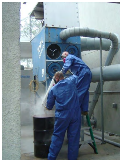
Figure 2. Maintenance technicians cleaning out the baghouse dust collector. Photo by NIOSH.
