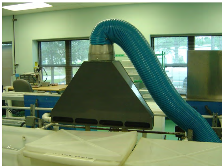
Figure 4. Local exhaust ventilation at the nitric acid passivation tank. Photo by NIOSH.
