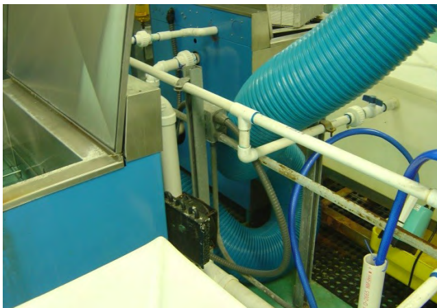
Figure 6. Excess duct in the nitric passivation area. Photo by NIOSH.
