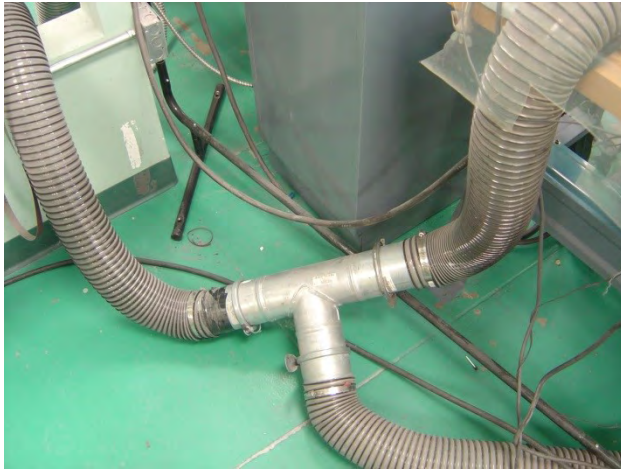
Figure 5. Local exhaust ventilation at the box polishing station. Photo by NIOSH.
