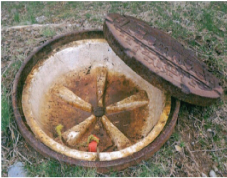
Figure 2. Manhole with rain guard intact. Photo by Veolia Environmental Service.
