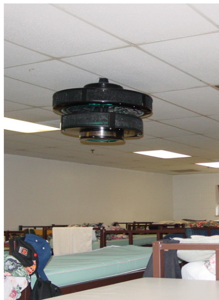
Figure 2. Typical upper-air UVGI installations: Left–Wall-mounted fixture with louvers installed in a health clinic; Right–Ceiling-mounted fixture with a fan installed in a homeless shelter.
