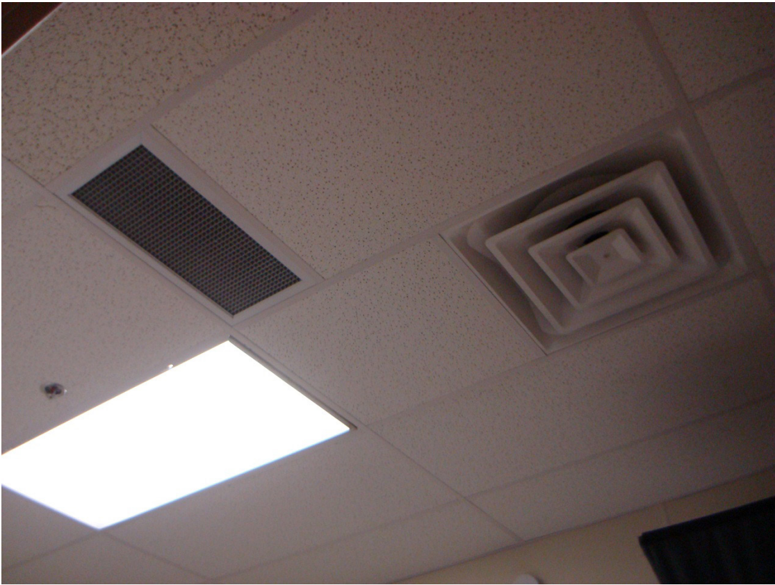
Figure 3. Supply vent and return grille in ceiling of family sleeping room #1 in the women's overnight facility. The close proximity of the supply to the return can result in short-circuiting of air, where supply air is immediately pulled into a return grille without providing any useful ventilation.
