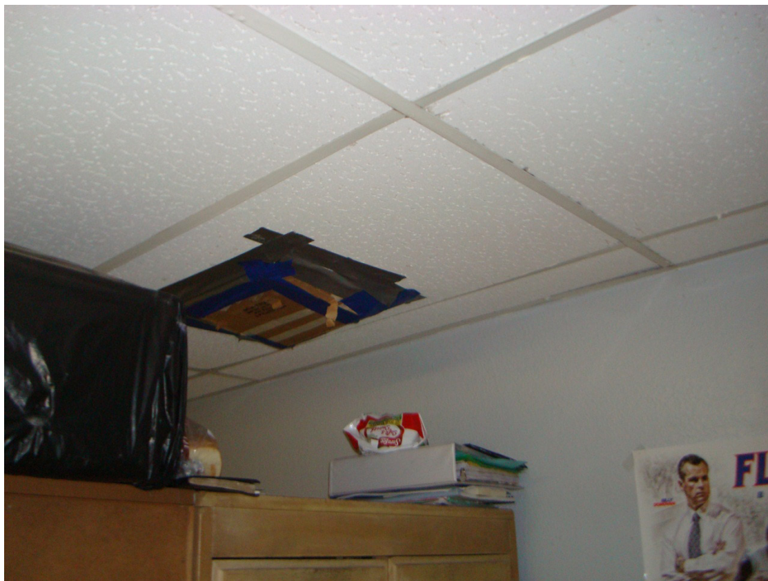
Figure 4. Supply vent covered with cardboard and tape in room #9 of the men's sleeping area.
