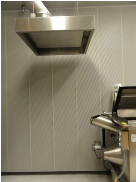
Figure 5. Canopy hood located approximately 3.75 feet above the breathing zone of the firearms inspector. Photo by NIOSH.
