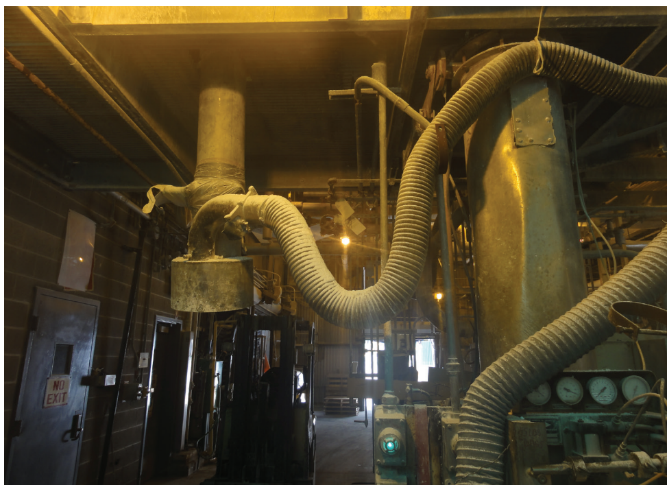
Figure 3. Excess ductwork to the super sack filling station. Photo by NIOSH.
