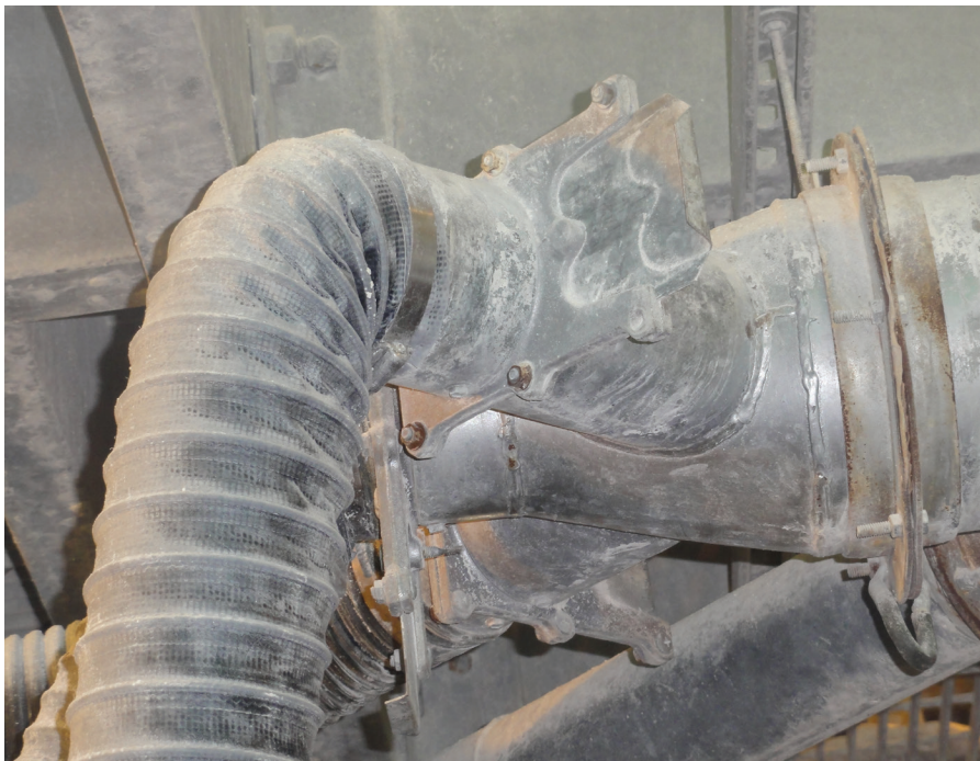
Figure 1. Pinched exhaust ductwork for the OTOS bag filling station. Photo by NIOSH.
