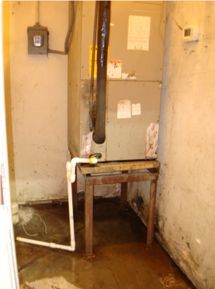
Figure 1. AHU-1 in the central mechanical room on the first floor of the shelter. The photograph shows standing water and apparent microbial growth due to condensate from the AHU leaking onto the floor of the mechanical room.
