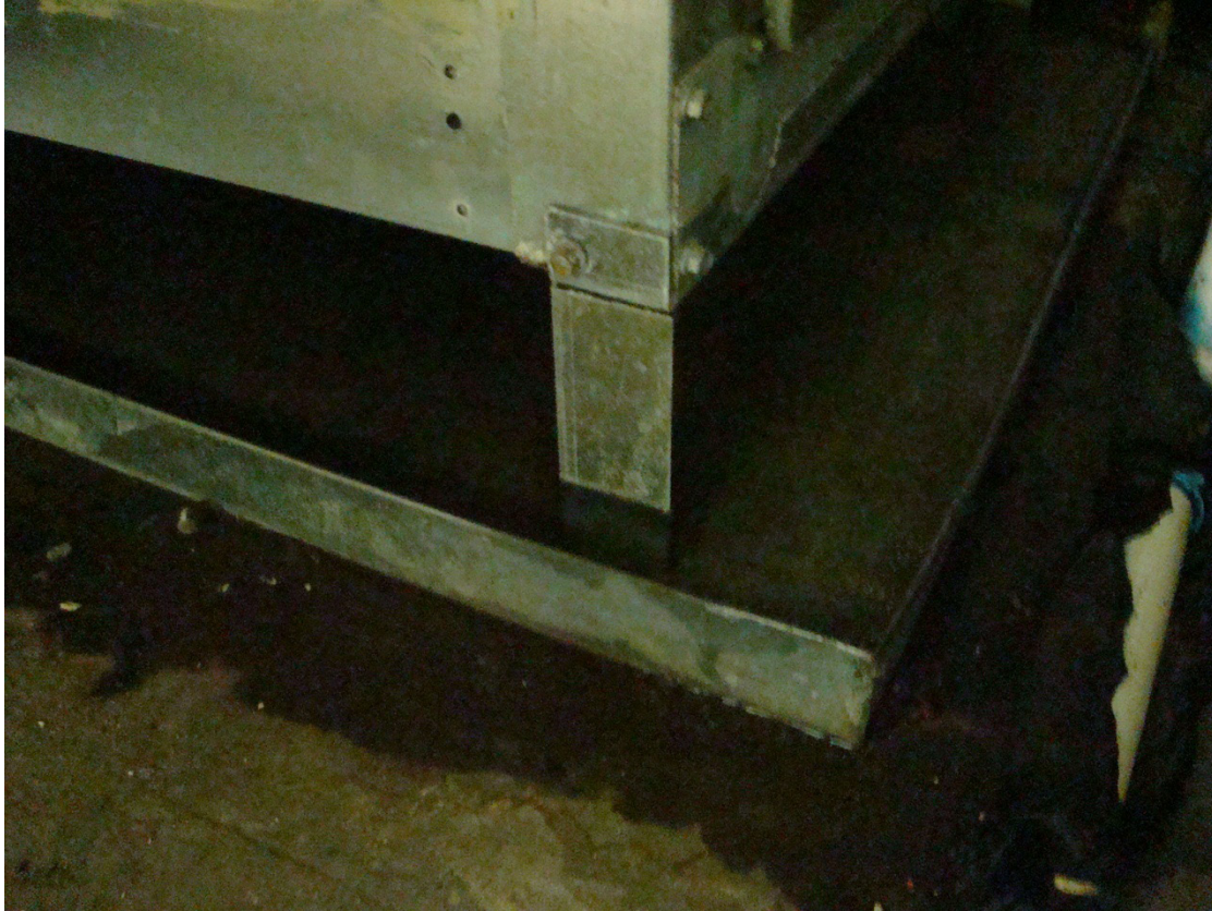
Figure 3. AHU-8 in the southeast corner mechanical room on the third floor of the shelter. The photograph shows a drain pan overflowing with condensate, which is covering the floor of the mechanical room.
