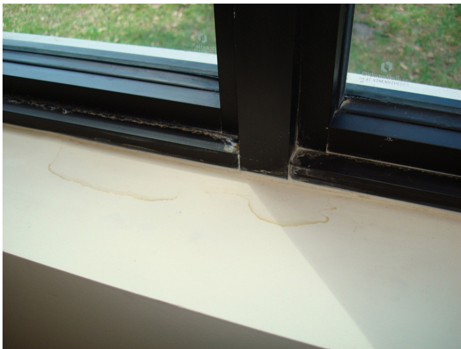
Figure 24. Water stains on window sill in Room 19, June 2011.
