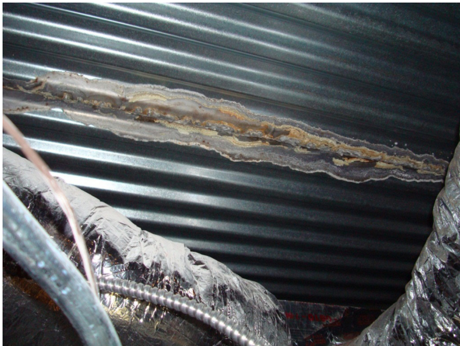
Figure 29. Rusty stain at a roof lap joint in ceiling plenum, June 2011.
