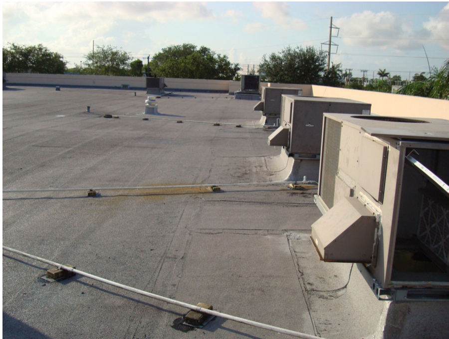
Figure 4. Roof-top air-handling units 1 (foreground) through 5 with condensate pipes that extend to roof drains, June 2011.
