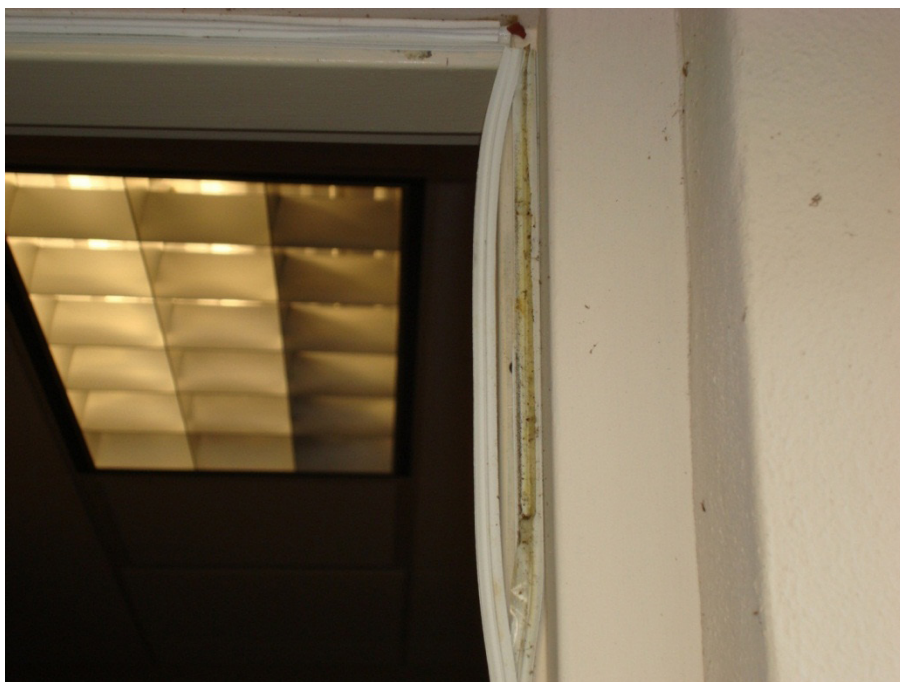
Figure 31. Ill-fitting weather stripping on Hall 5 exterior door frame, June 2011.
