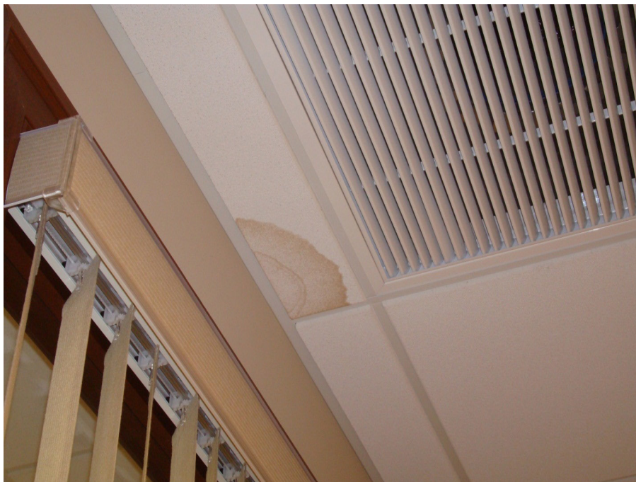
Figure 19. Ceiling stain in Room 23, June 2011.
