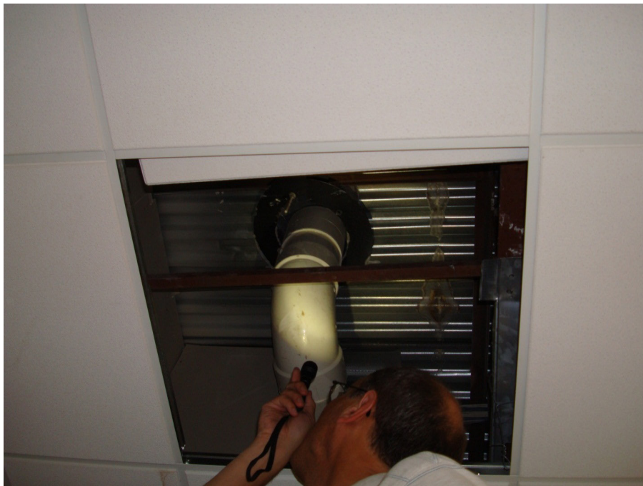
Figure 22. Roof drain above ceiling stain in Room 37 (kitchen), June 2011.
