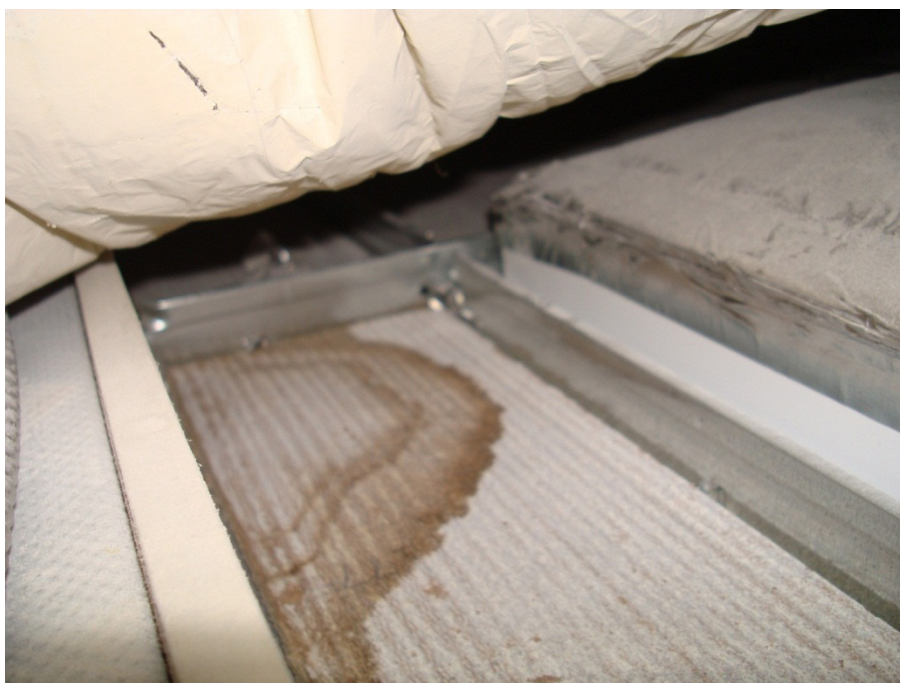
Figure 20. Top of stained ceiling tile in Room 23, June 2011.
