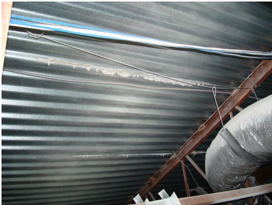
Figure 27. Roof lap joints inside ceiling plenum, June 2011.
