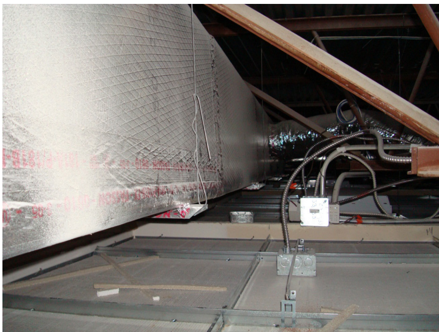
Figure 9. HVAC main trunk line, June 2011.
