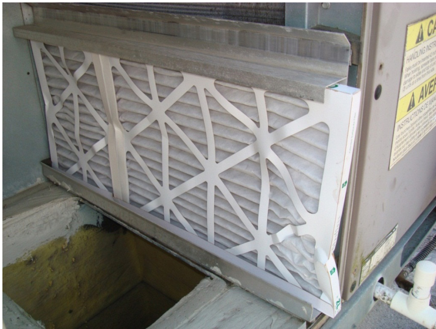
Figure 35. Oversized filter in AHU-2, June 2011.
