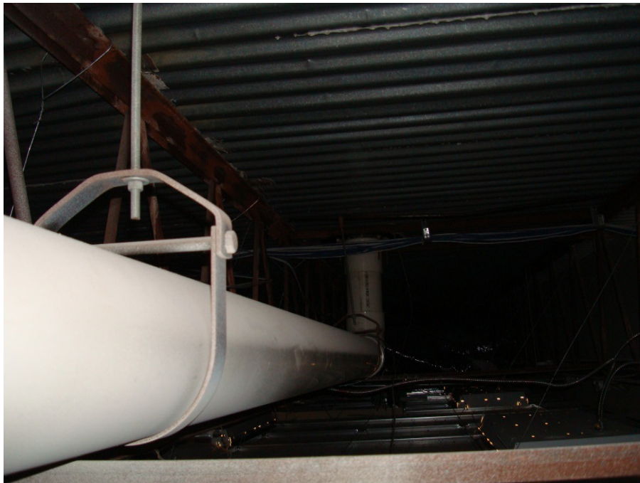
Figure 5. Roof drainpipe inside ceiling plenum, June 2011.
