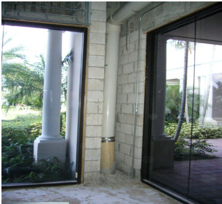
Figure 6. Roof drainpipe dropped through the exterior wall (exposed during 2006-7 renovation) into the ground, October 2006 (picture courtesy of building manager).
