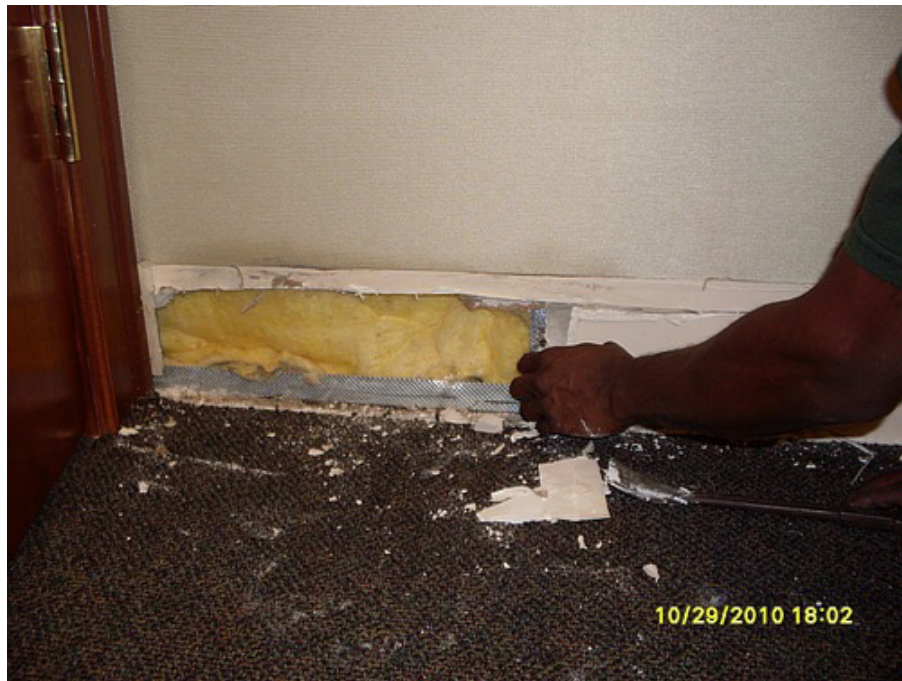
Figure 14. Suspect mold-damaged drywall removed in Room 3 at base of wall shared with Hall 5, October 2010 (picture courtesy of building manager).
