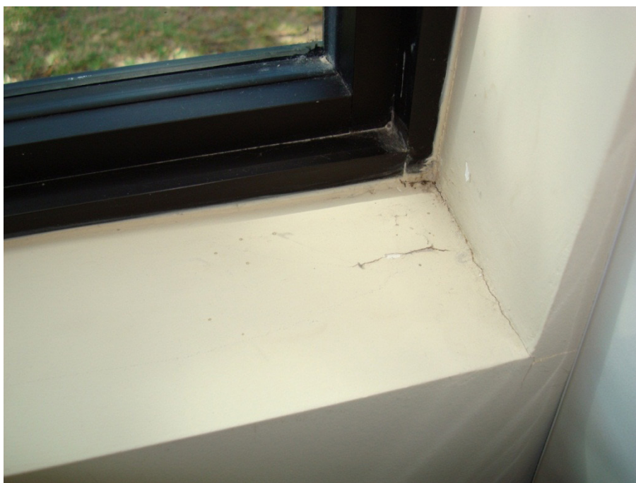
Figure 25. Blistered paint on window sill in Room 19, June 2011.
