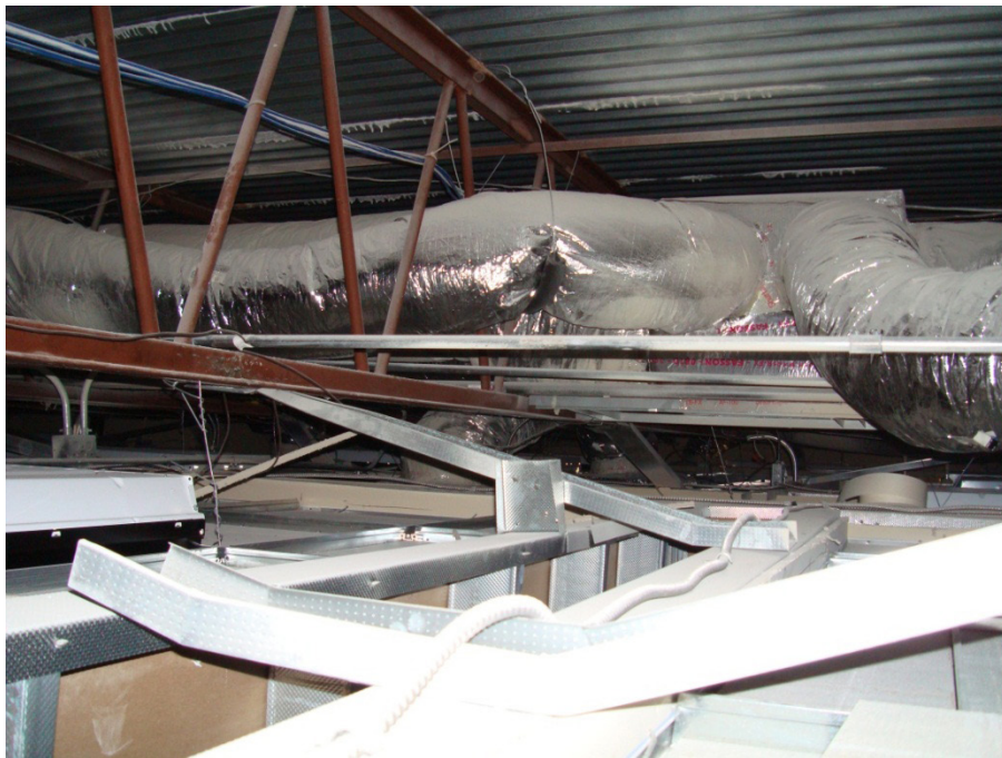
Figure 10. HVAC main trunk line with multiple flexible ducts attached, June 2011.
