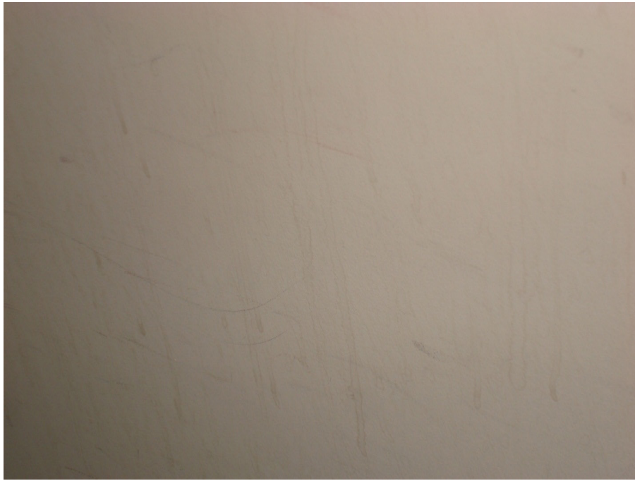
Figure 26. Vertical water marks on wall under window in Hall 11, June 2011.
