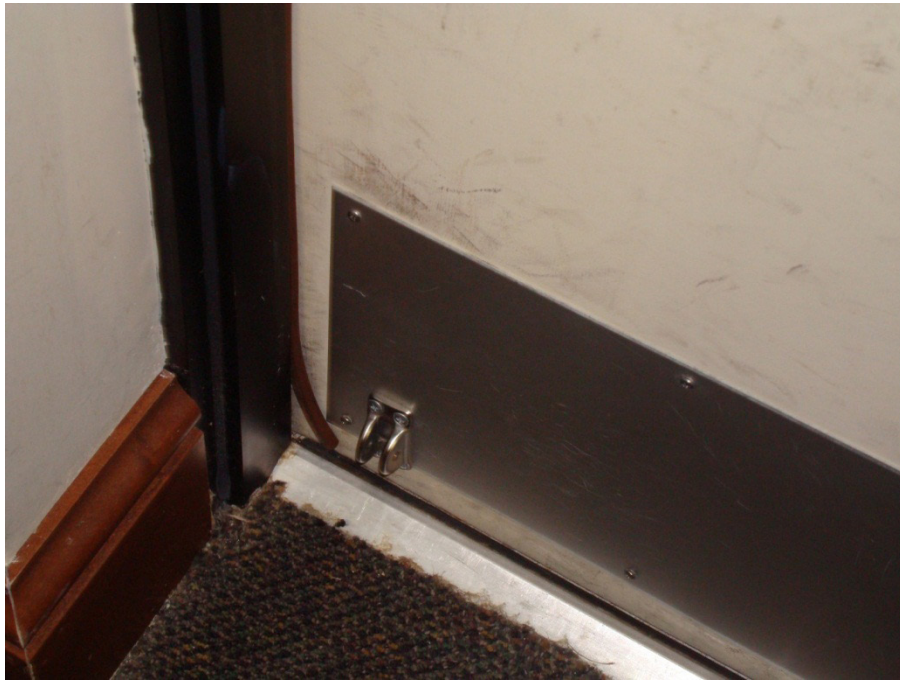
Figure 32. Ill-fitting weather stripping on door frame in Hall 5, June 2011.
