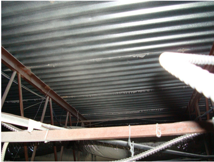
Figure 28. Roof lap joints inside ceiling plenum, June 2011.
