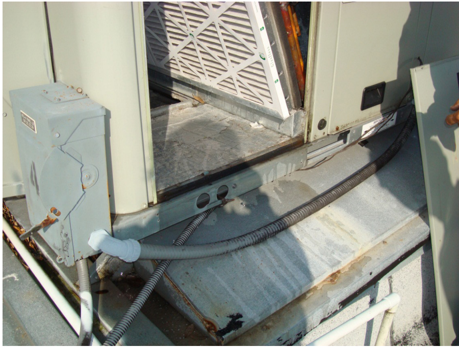
Figure 36. Water dripping into AHU-4 filter housing base and outside/return air mixing plenum, June 2011.
