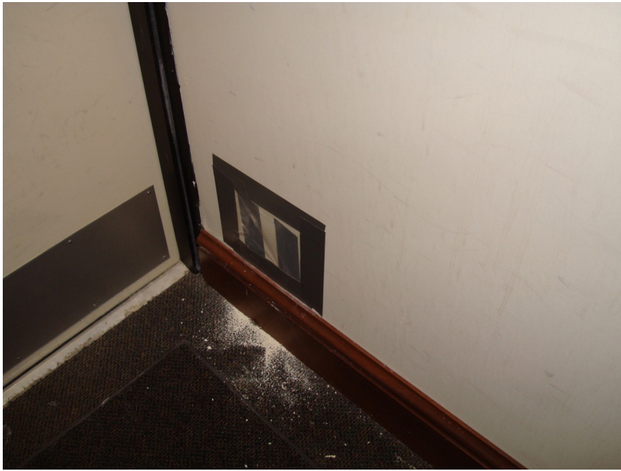
Figure 12. Wall cavity inspection hole after sealing with tape in Hall 11 wall shared with Room 10, June 2011.
