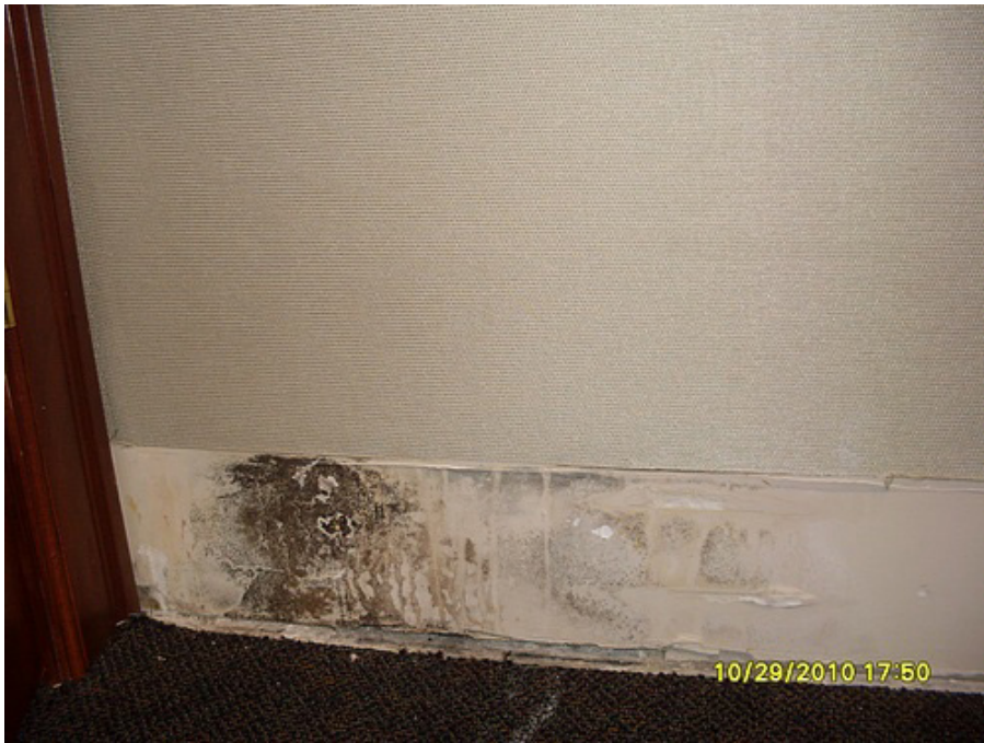
Figure 13. Suspect mold in Room 3 at base of wall shared with Hall 5, October 2010 (picture courtesy of building manager).
