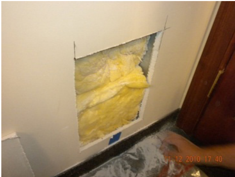
Figure 17. Wall cavity inspection inside Hall 5 wall shared with Room 3, November 2010 (picture courtesy of building manager).
