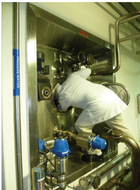
Figure 2. Equipment inspector makes a partial entry into a cream tank.
