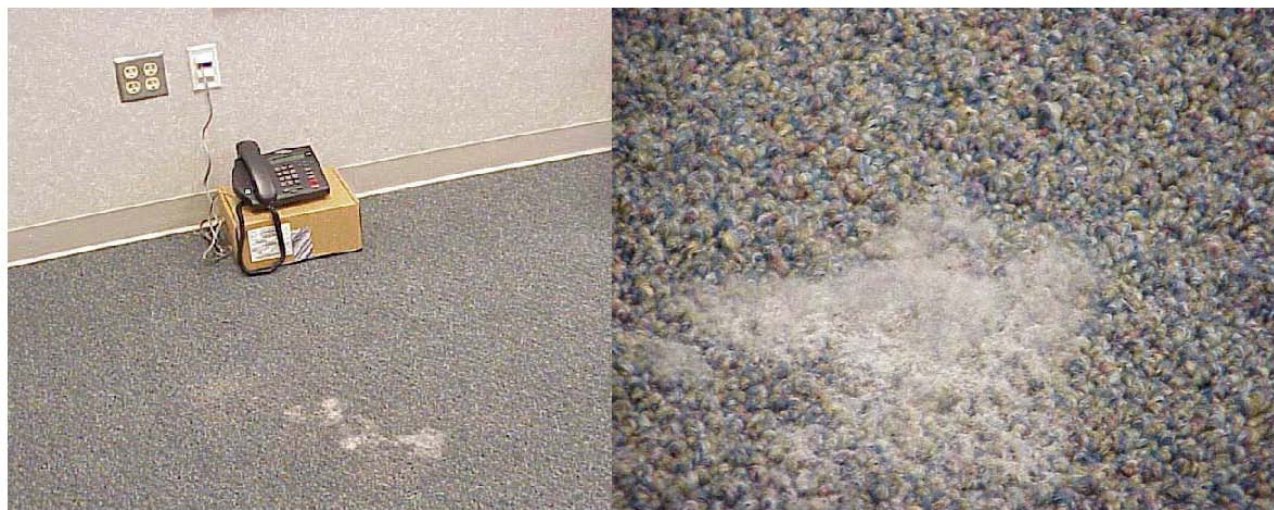
Figure 2. Visible mold on carpet in classroom 625, August 10, 2005 (courtesy of building occupant)
