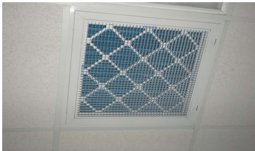
INSTALLATION OF NEW FILTER BOXES IN CLASSROOM
