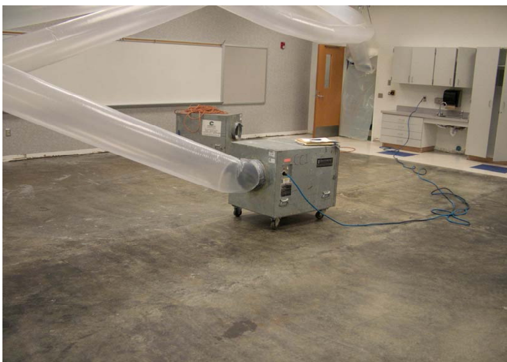
Typical Classroom Containment & Isolation
