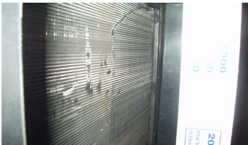
CLEANED COILS
