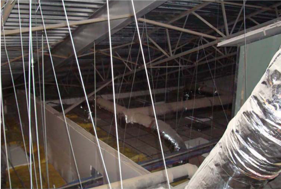
Figure 14. Plenum above classroom ceiling, showing ductwork and dust, July 2009.
