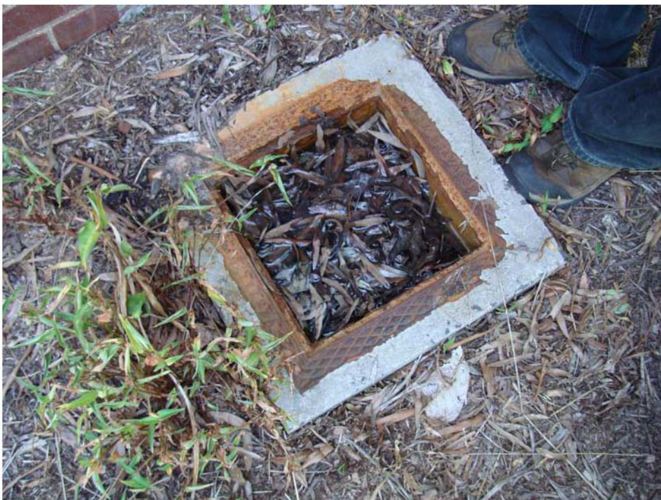
Figure 9. Blocked storm drain outside of the media center, July 2009.
