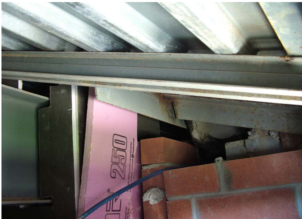
As Found Soffit Air Leaks
