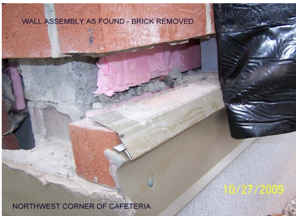
As Found Roof Flashing
