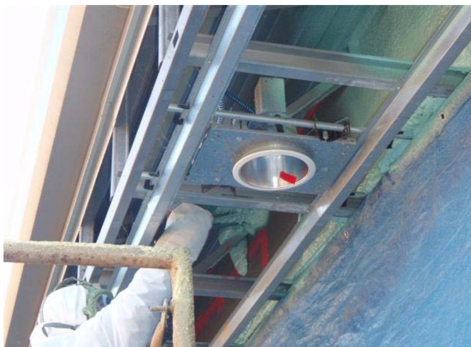
Soffit Sealing
