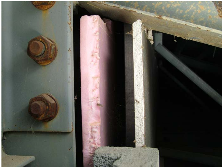
As Found Soffit Air Leaks
