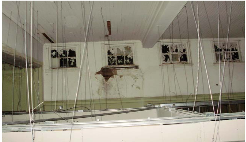
REMOVAL OF CEILING TILES
