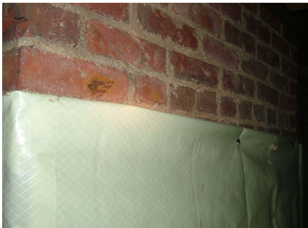
Crawl Space Vapor Barrier
