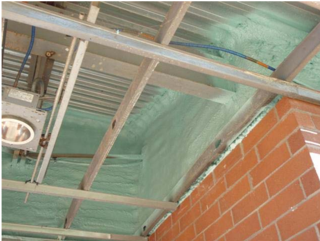
Soffit Sealing
