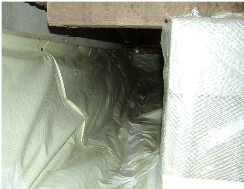
Crawl Space Vapor Barrier
