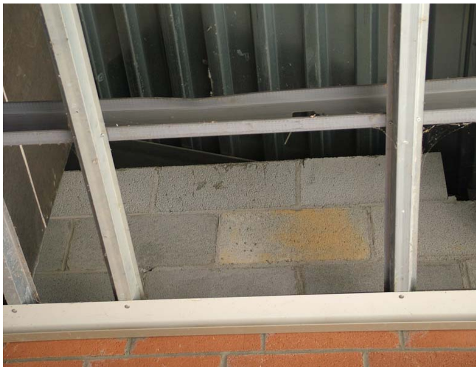
As Found Soffit Air Leaks
