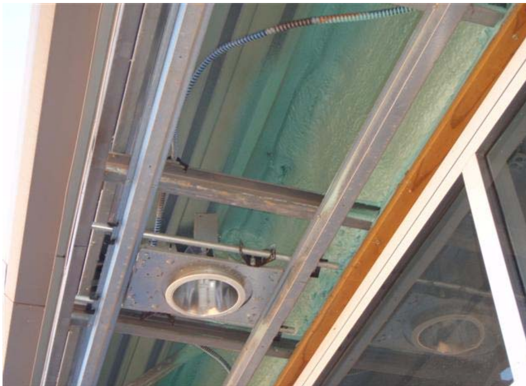
Soffit Sealing
