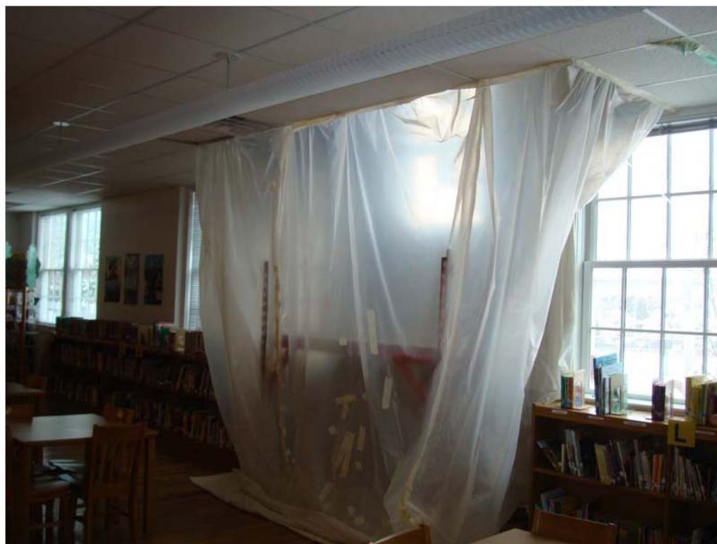
Figure 23. Media center, showing temporary containment barrier for installation of exterior door, March 2010.
