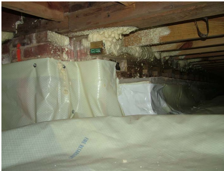
Crawl Space Vapor Barrier
