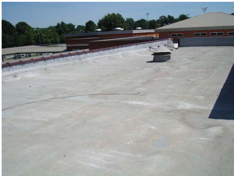
Figure 11. Foam roof over media center wing, July 14, 2009
