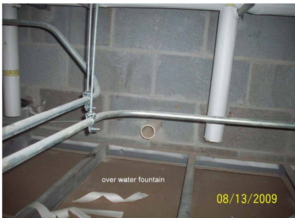
Open Plumbing Vent Lines
