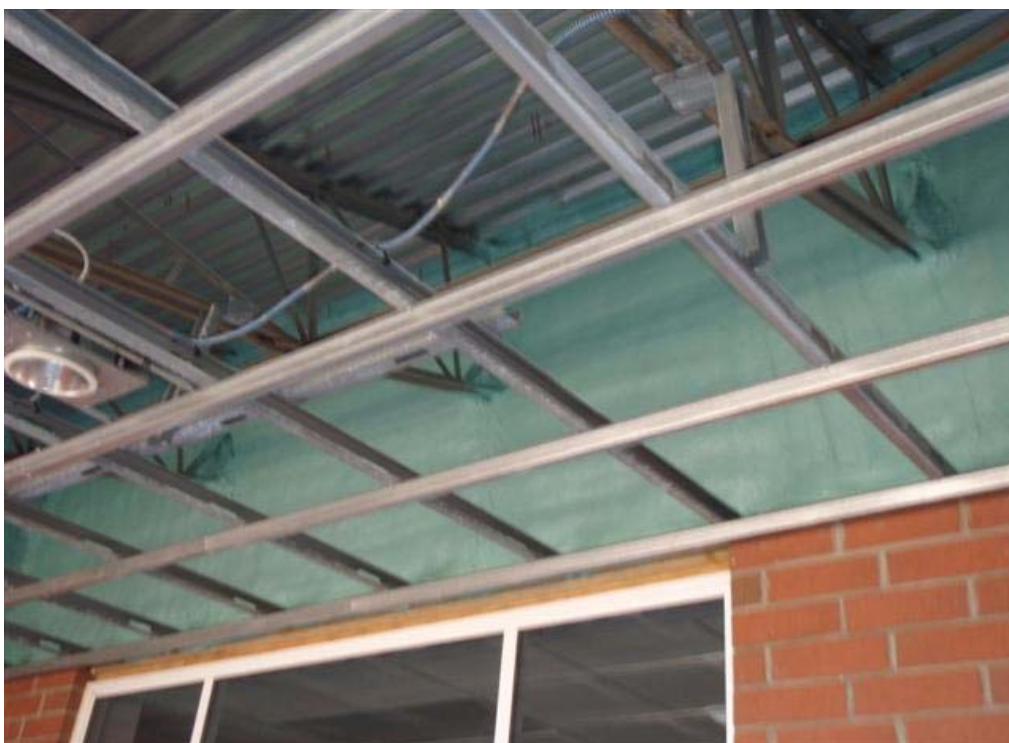
Soffit Sealing
