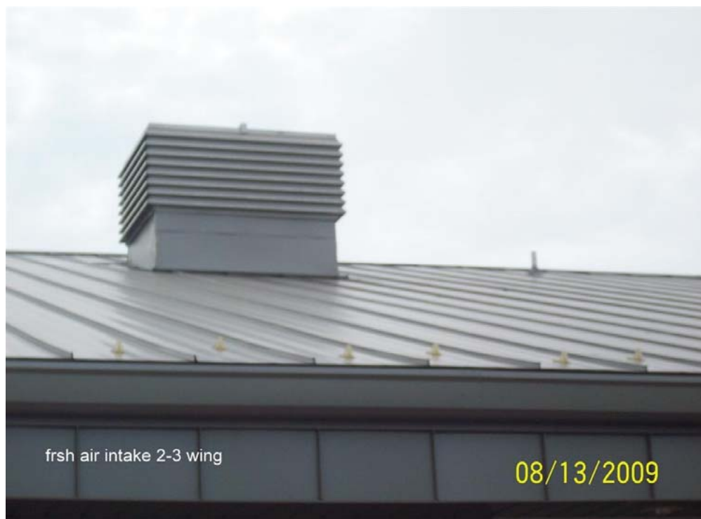
Vent Through Roof And OA Inlet
