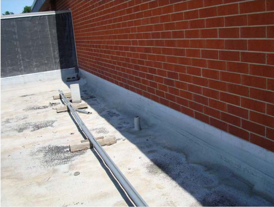
Figure 10. Foam roof adjacent to gym, July 2009.
