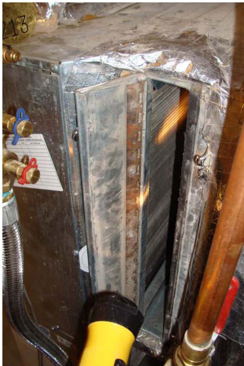
Figure 15. Coils in HVAC air handlers, showing dust and possible mold contamination, July 2009.
