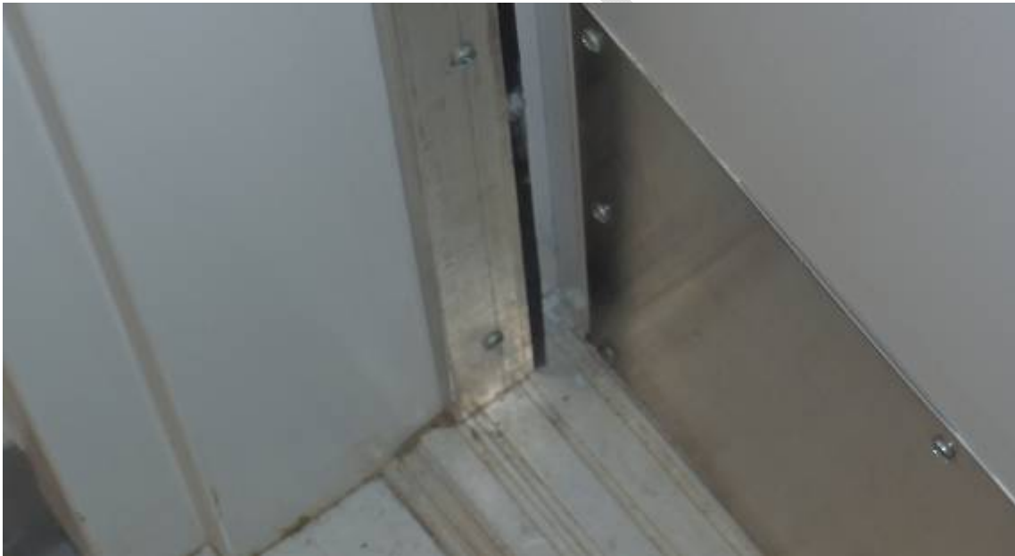
Figure 9 – Classroom 521 door showing 1/2" gap when door not physically pulled shut
