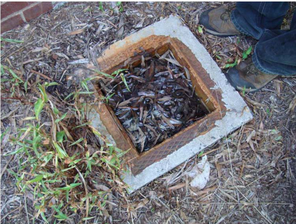
Figure 9. Blocked storm drain outside of the media center, July 14, 2009
