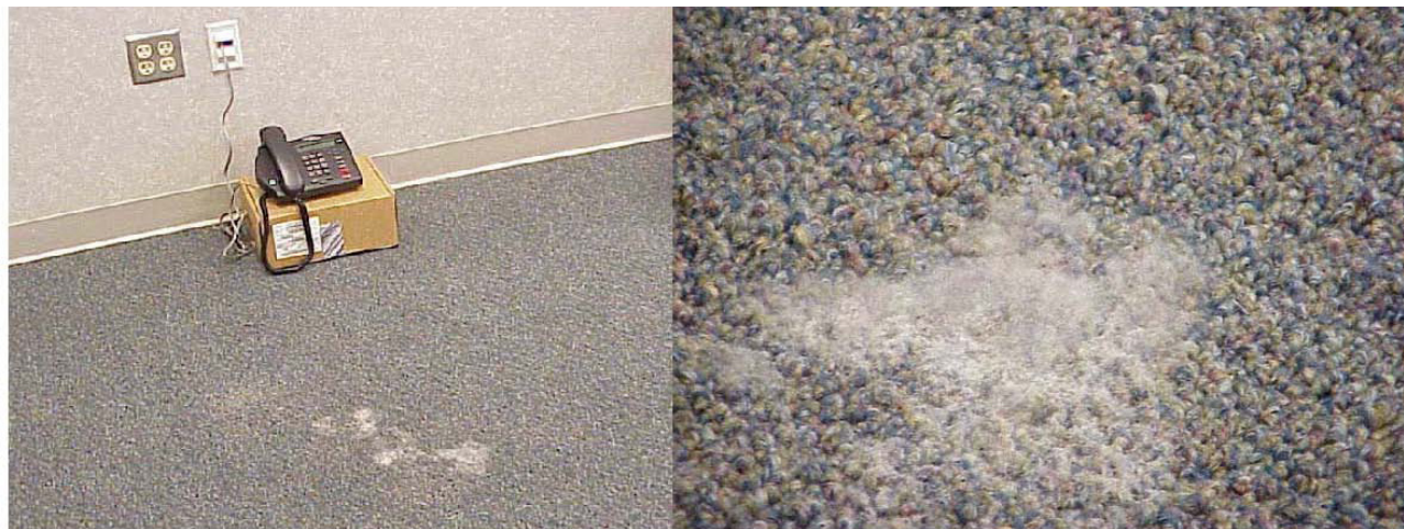
Figure 2. Visible mold on carpet in a classroom (room 625), August 2005 (courtesy of building occupant).
