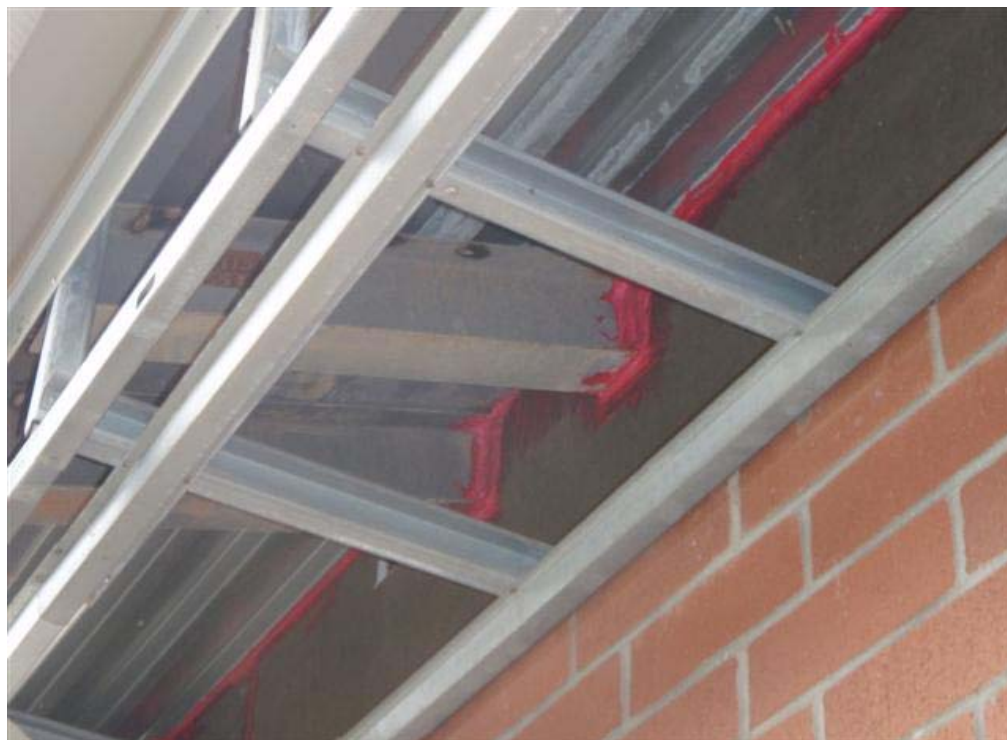
Soffit Sealing
