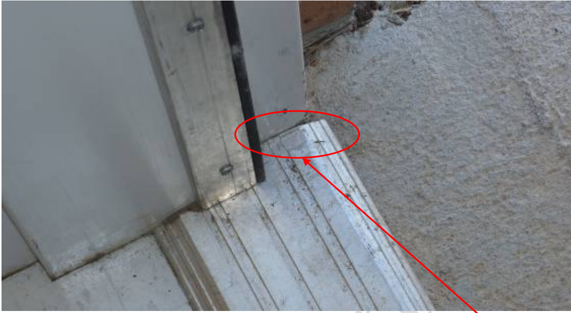
Figure 8 – Outside door of classroom 521 dragging on threshold
