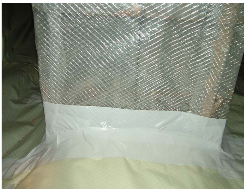
Crawl Space Vapor Barrier
