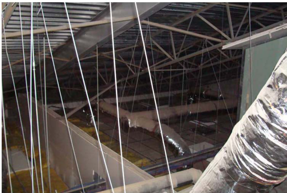
Figure 14. Dust on classroom ceilings and ducts in plenum, July 16, 2009
