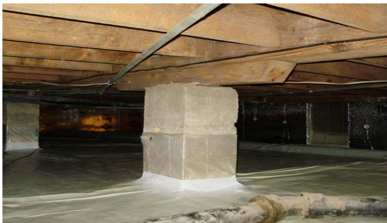
CLEANED FLOOR SYSTEM AND INSTALLED VAPOR BARRIER
