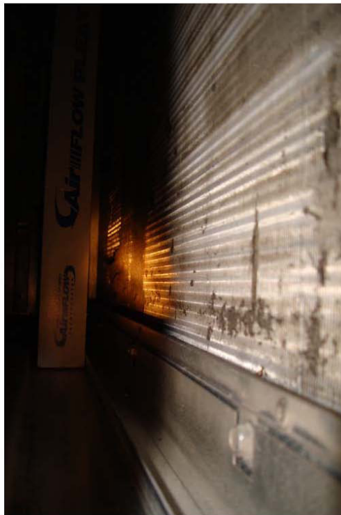
Figure 15. Coils in HVAC air handlers, showing dust and possible mold contamination, July 2009.
