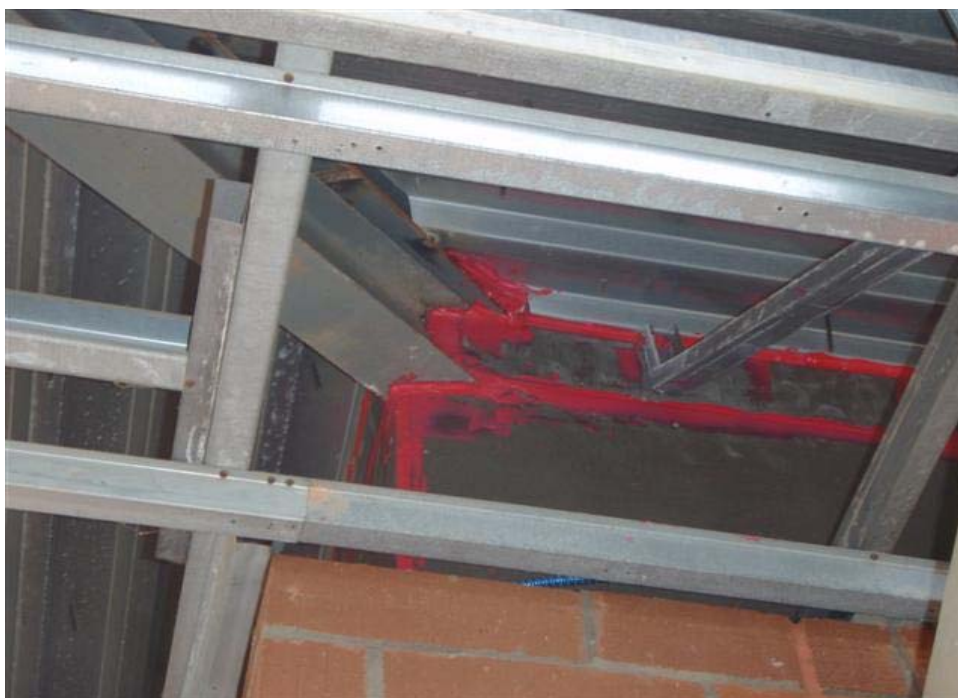
Soffit Sealing
