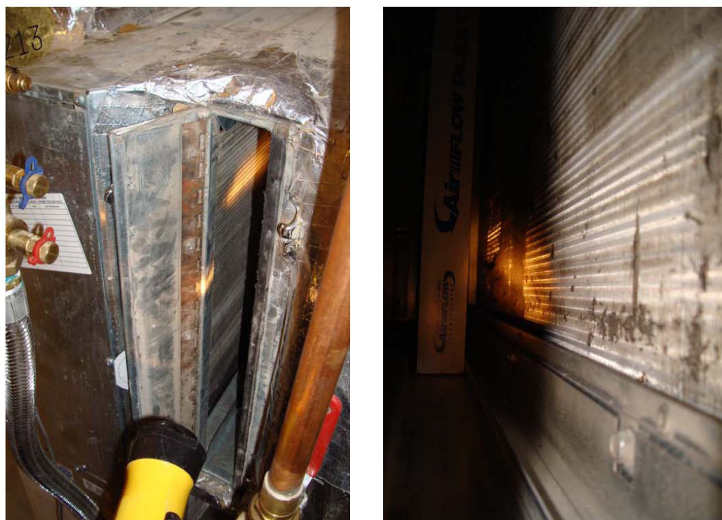
Figure 15. Coils for HVAC handlers showing dust and possible mold contamination , July 16, 2009
