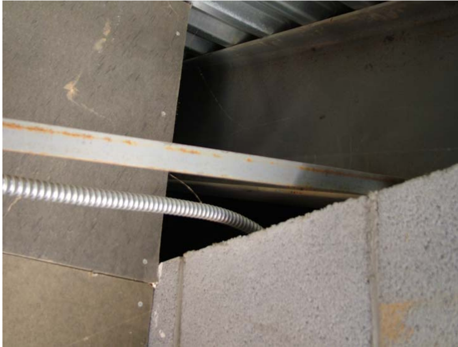
As Found Soffit Air Leaks
