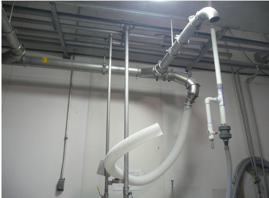
Figure 1. Disconnected and uncapped local exhaust ventilation duct on line one.
