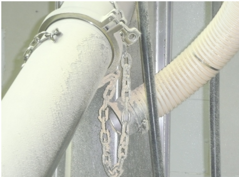
Figure 2. Disconnected and uncapped local exhaust ventilation duct on line one.
