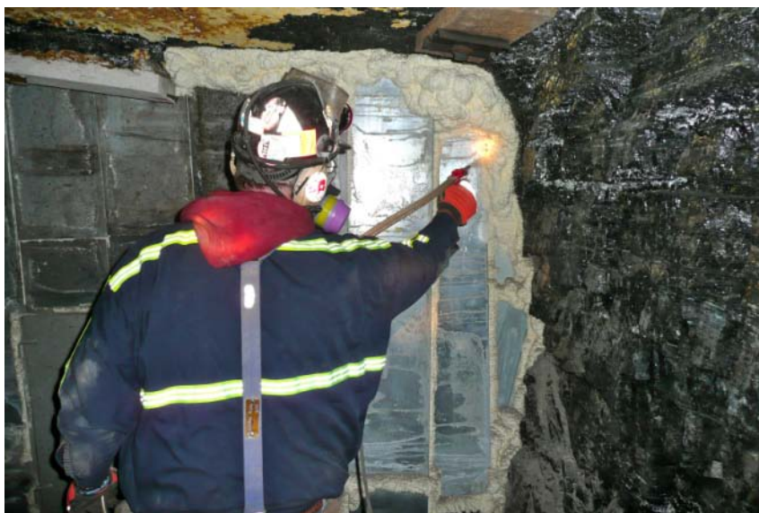
Figure 1. Applying polyurethane foam to a steel ventilation stopping.
