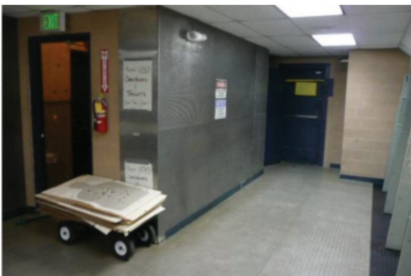
Figure 2. Perforated metal wall plenum near the firing range entry door.
