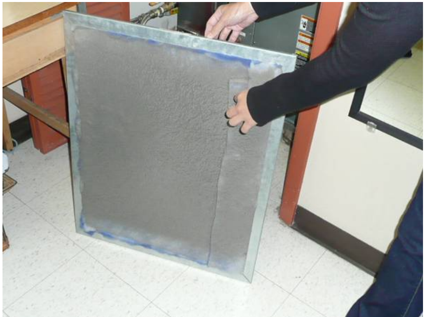
Figure 7. Dirty air filter removed from the HVAC system made of pieces of roll-type low-efficiency prefilter material.
