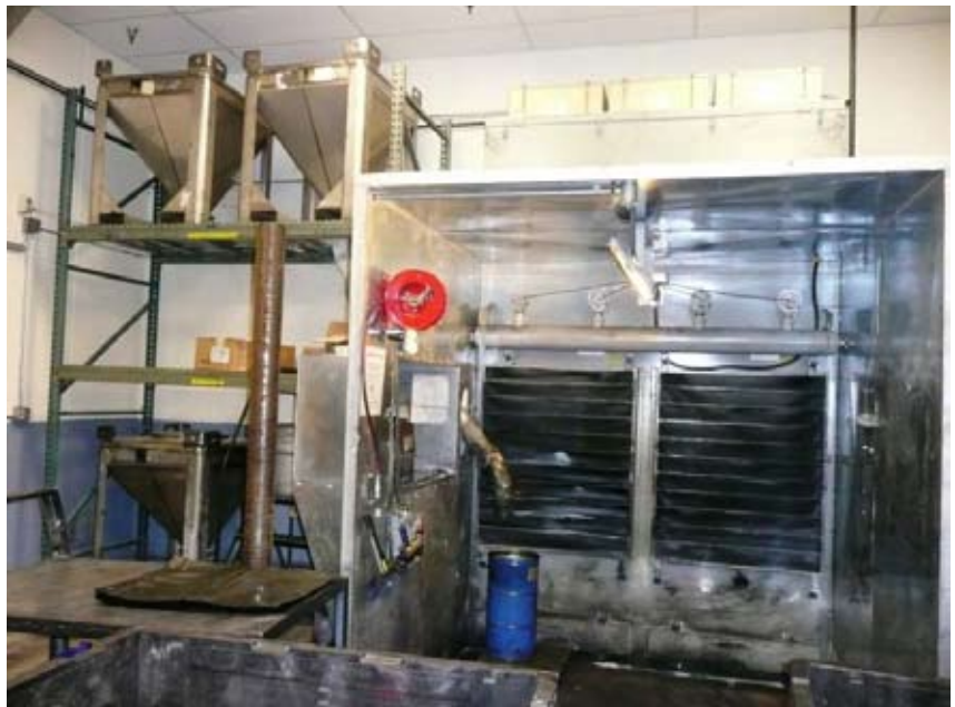
Figure 5. Semiventilated downdraft booth installed in the kitting room – September 2009.
