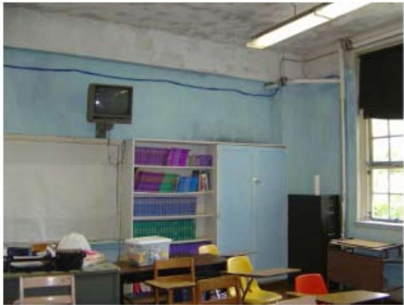
Figure 2. Picture of fourth floor classroom wall and ceiling showing active mold growth at AFSHS
