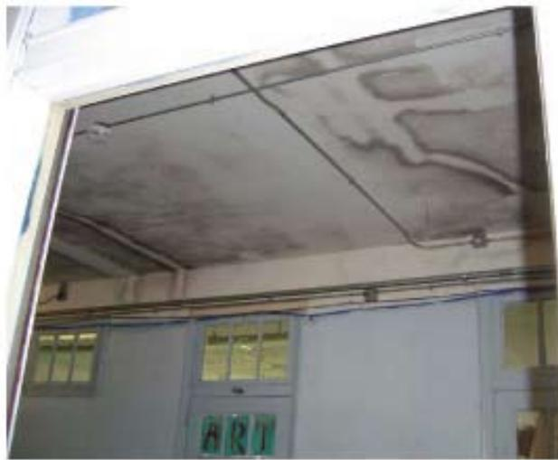
Figure 1. Picture of mold growing along fourth floor hallway ceiling at AFSHS
