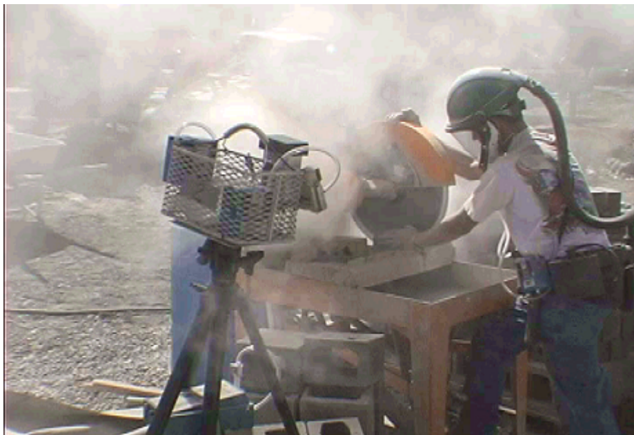
Figure 1. Video snapshot during dry sawing of brick. A powered air purifying respirator is being worn by the worker. An air sampling station is located on a tripod to the left of the worker.
