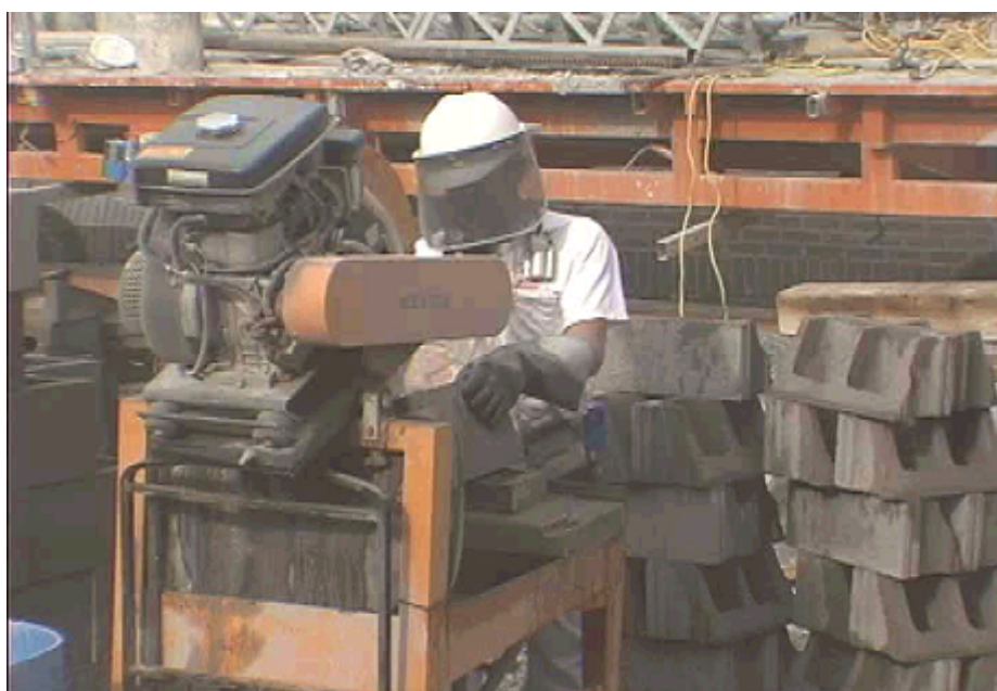
Figure 2. Video snapshot during wet sawing of block. A simple face shield is being worn by the worker for splash protection. Note the personal impactor air sampler on the left lapel of the worker.
