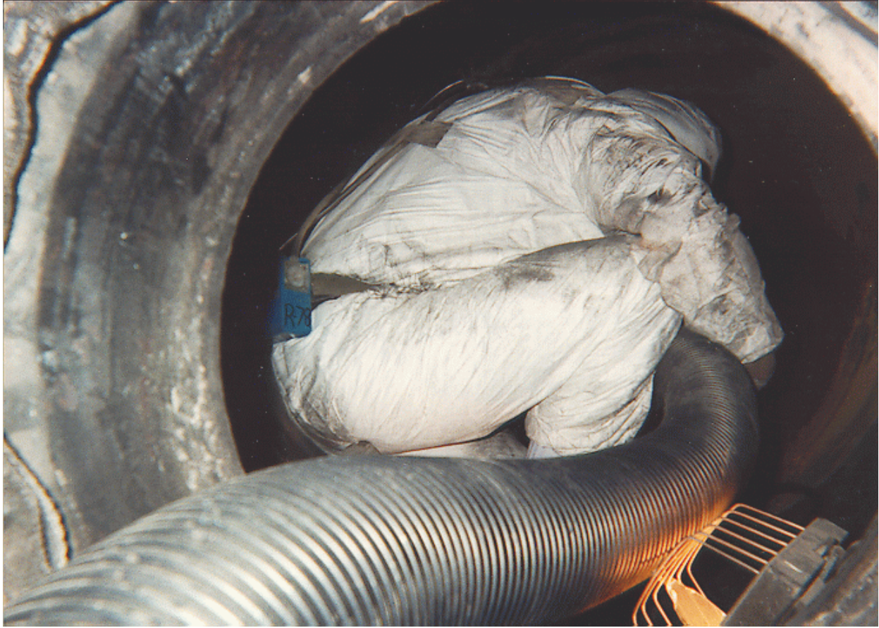
Figure 3. Worker cleaning inside the boiler with ventilation duct.
