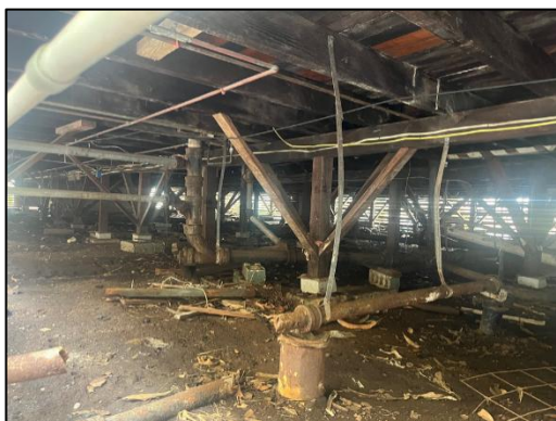
Photo 3: Post and pier foundation. (Courtesy of NIOSH)
