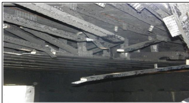
Photo 5 and 6: Lightweight parallel chord trusses. Left shows the truss as new and the other shows how the truss loses structural integrity after less than 5 minutes of fire exposure. (Courtesy of FRSI)
