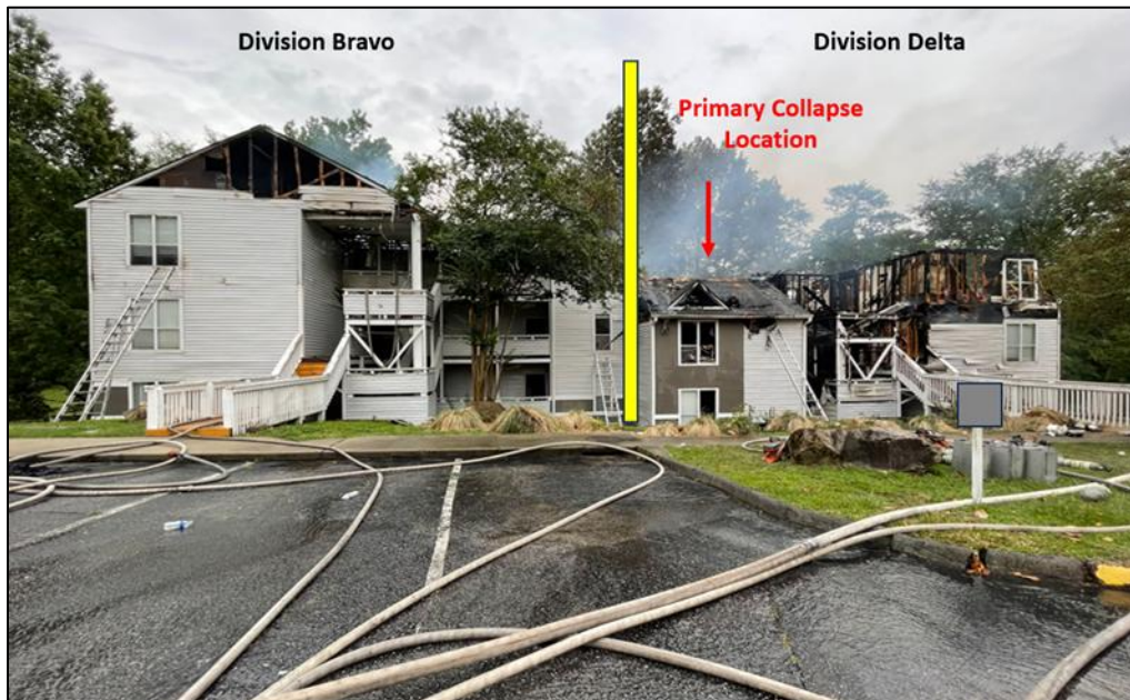
Photo 3: Division Bravo (left) and division Delta (right) separation. (Prepared by NIOSH)
