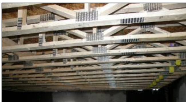
Photo 5 and 6: Lightweight parallel chord trusses. Left shows the truss as new and the other shows how the truss loses structural integrity after less than 5 minutes of fire exposure. (Courtesy of FRSI)
