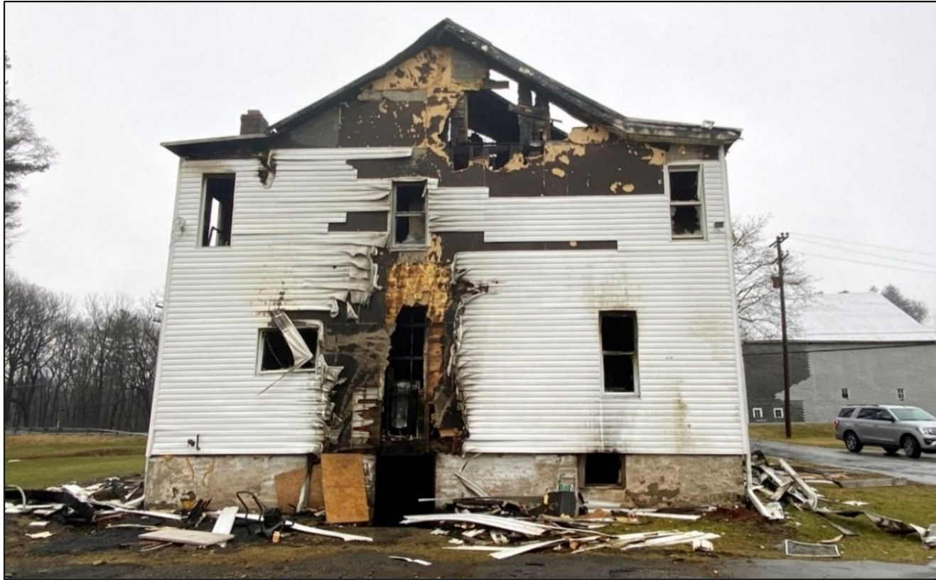
Side Charlie. The exterior door to the rear cellar is visible. The fire extension pathway from the cellar to the top half story is clearly visible. (Courtesy of NIOSH)
