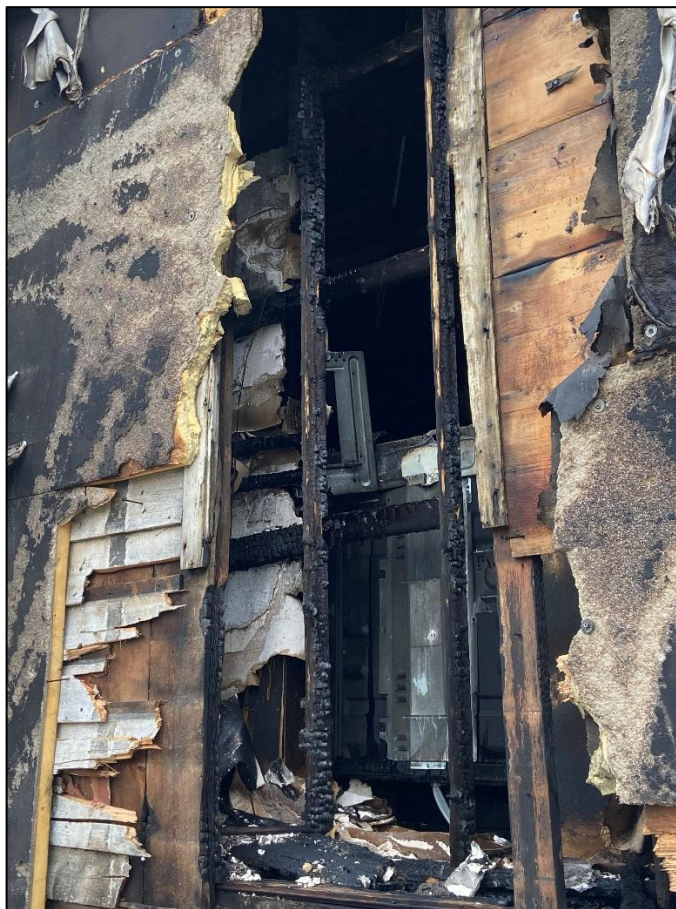
Photo 6. First floor Side Charlie wall construction showing original plank wall and new interior wall creating a void space. ( Courtesy of NIOSH )
