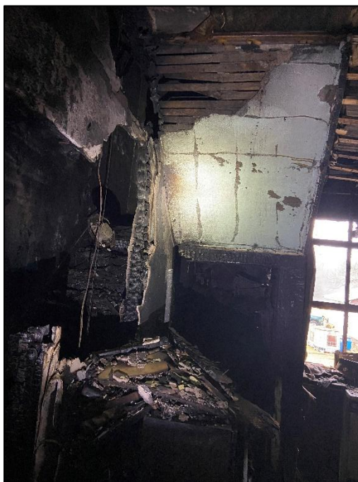
Photo 11. Rear stairs, showing the flow path from the rear cellar, to the first floor, to the second floor (Side Charlie).
