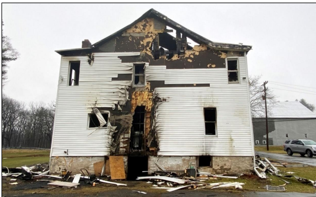
Photo 3. Side Charlie. The exterior door to the rear cellar is visible. The fire extension pathway from the cellar to the top half story is clearly visible. (Courtesy of NIOSH)
