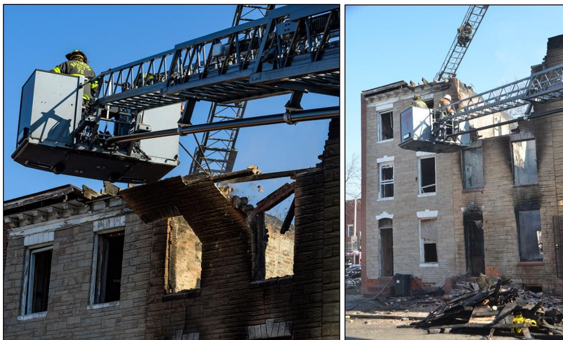
Photo 5 (left) and Photo 6 (right). Tower 1 firefighters were using 8-foot and 10-foot hooks to remove large sections of the Side Alpha wall. Contractors had made cuts in the Side Alpha wall with a circular saw.
