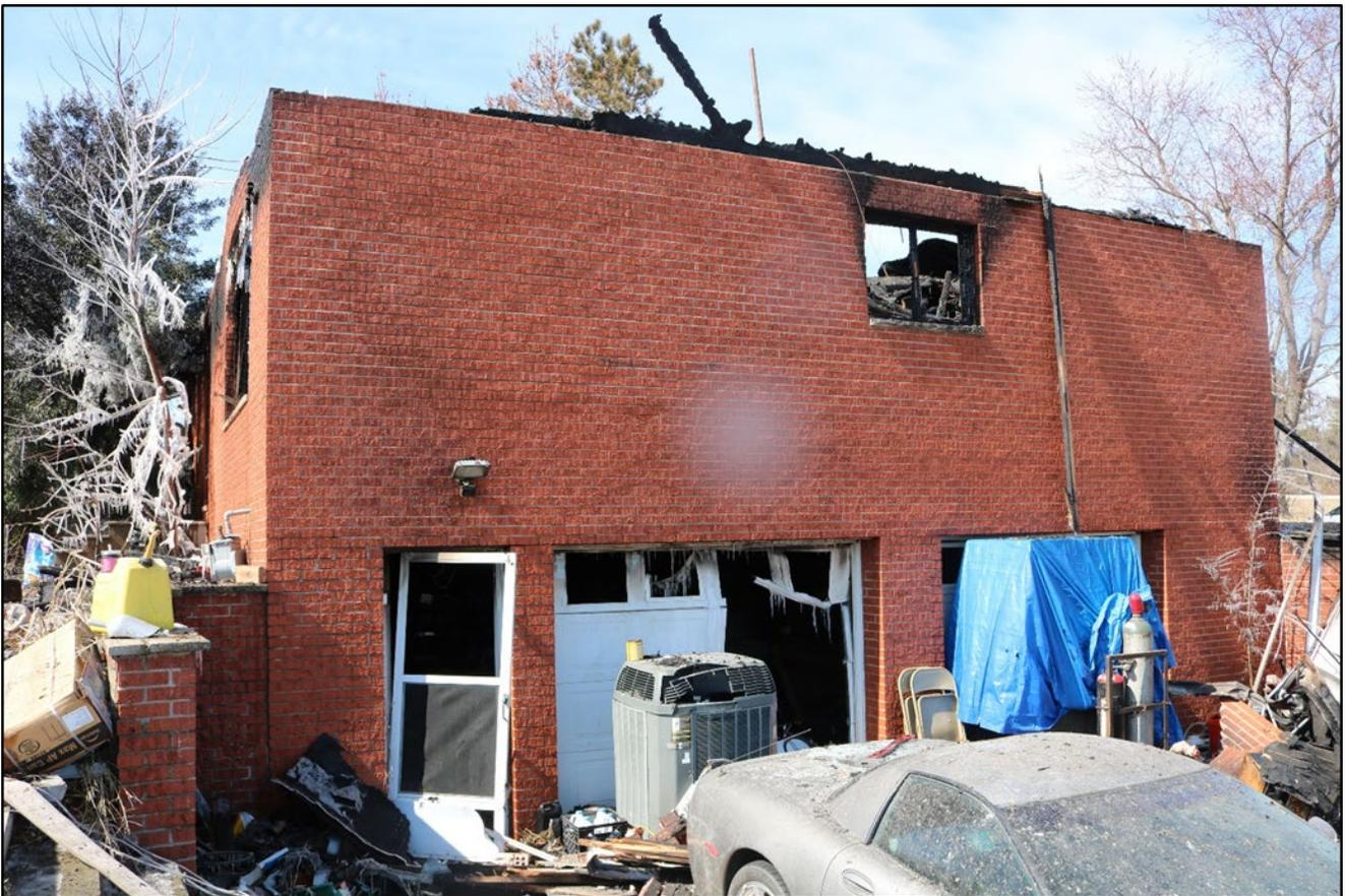
**Photo 5. Side Bravo showing below grade man door on the Side Bravo/Charlie corner, as well as the left and right garage doors. The photo was taken after the brick gable had collapsed. The right side of the garage door has been cut open.**
