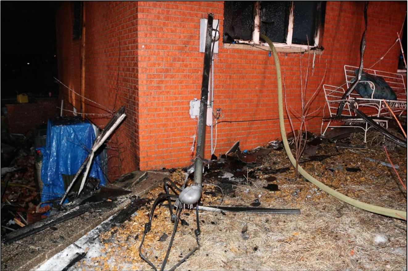
**Photo 6: Downed power line entering the home at the Side Alpha/Bravo corner.**
