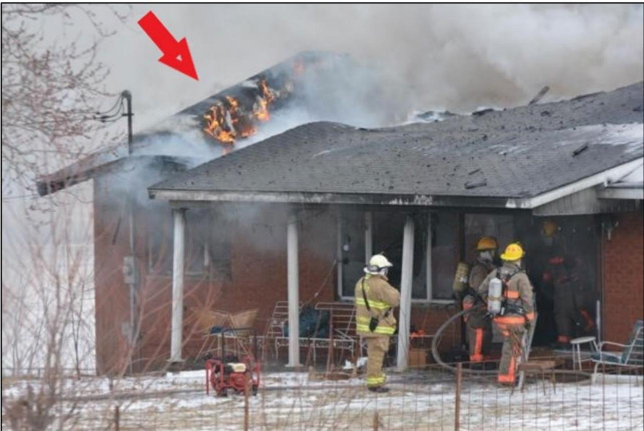
**Photo 3. Firefighters conducting interior operations thru the front door even though approximately 45 to 50% of the roof had collapsed into the 1<sup>st</sup> floor. Red arrow indicates the end of the bricked gable rafter that eventually collapsed onto the driveway on Side Bravo.**
