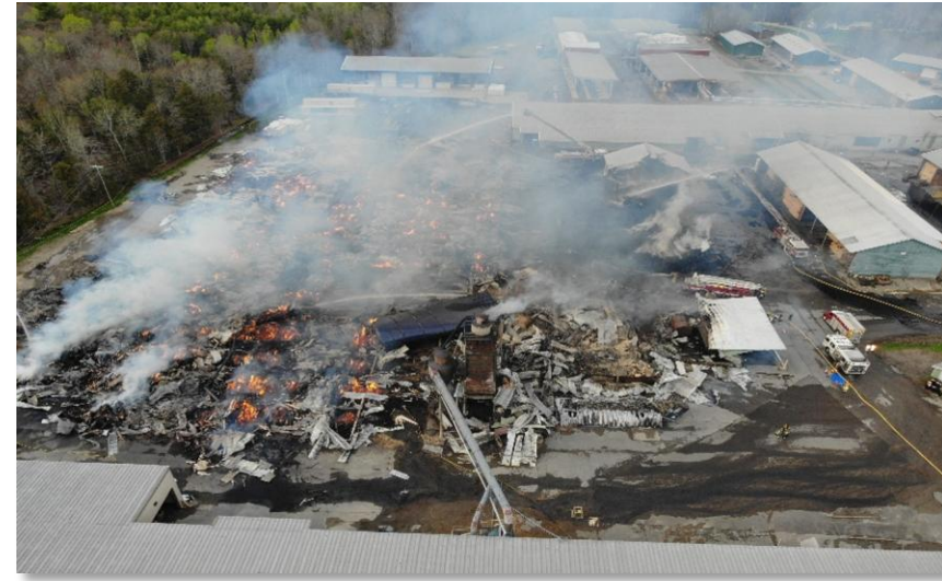
Aerial view of incident from Side Bravo of incident silo, post-explosion. (Source: State Fire Marshal's Office)
