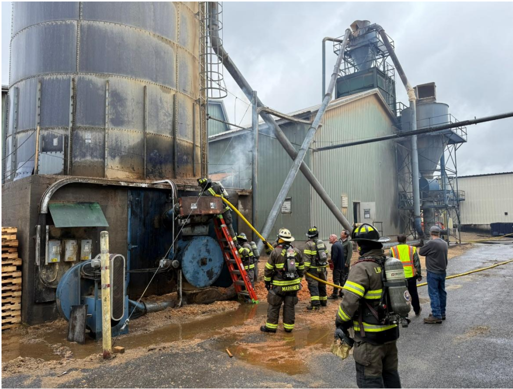
Image 11. Lieutenant 40 flowing water into the blower on Side Charlie. (Source: Fire department)
