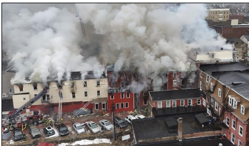
Photo 1: View of structure, Side Bravo. (Courtesy of the fire department)
