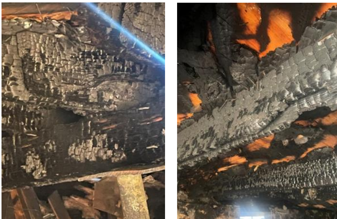
Photo 5 and 6: View of joist charring. (Courtesy of the fire department)
