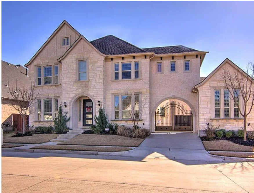
Photo 2: View of structure, pre-incident. (Courtesy of the fire department)
