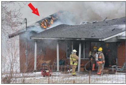
Firefighters conducting interior operations thru the front door even though approximately 45 to 50% of the roof had collapsed into the 1st floor. Red arrow indicates the end of the bricked gable rafter that eventually collapsed onto the driveway on Side Bravo. Photo taken from Side Alpha looking toward Side Bravo.
