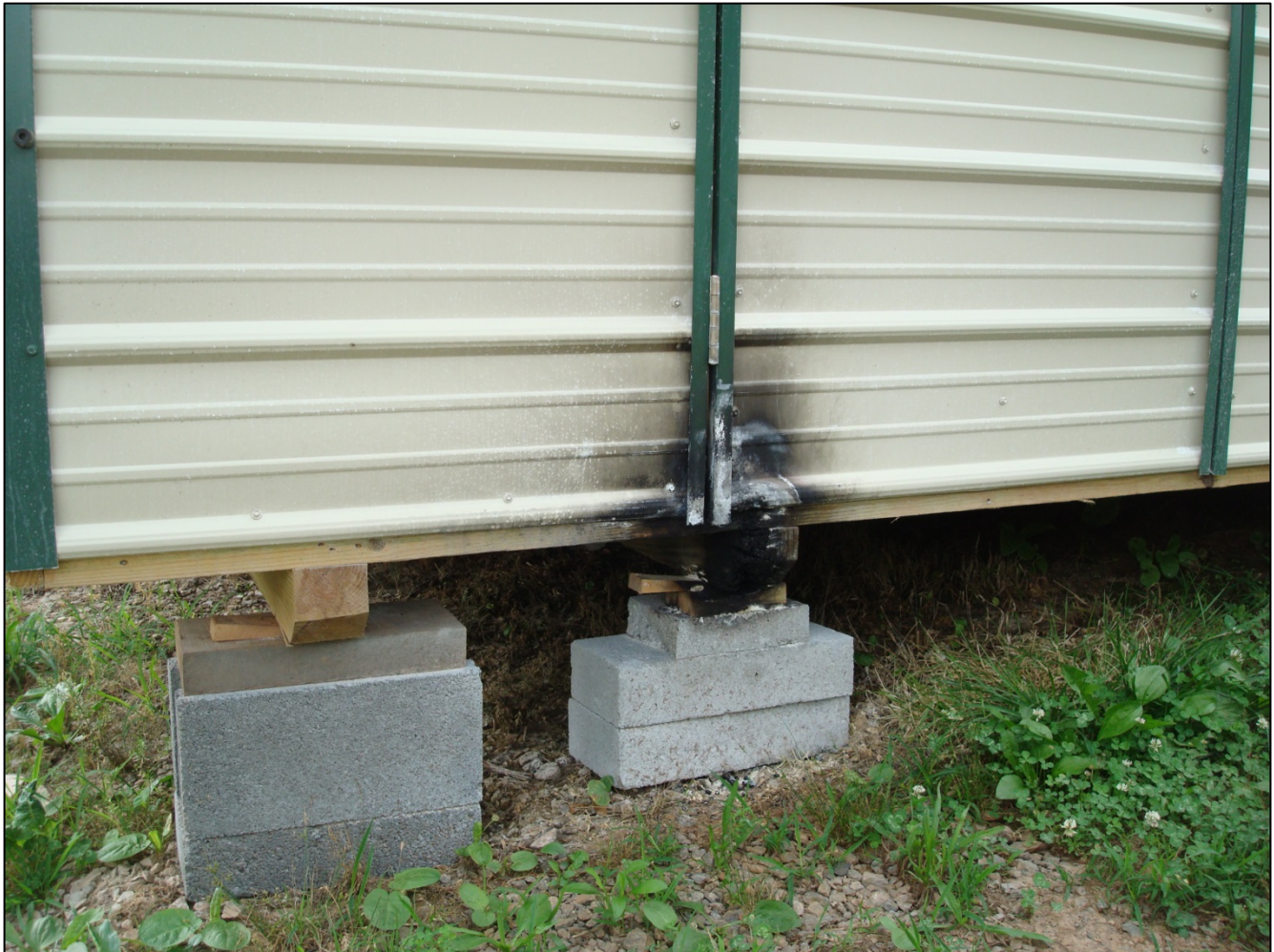
Photo 2. Close-up of metal storage building showing the support structure and location where electrical current went to ground, causing wooden supports to catch fire.
