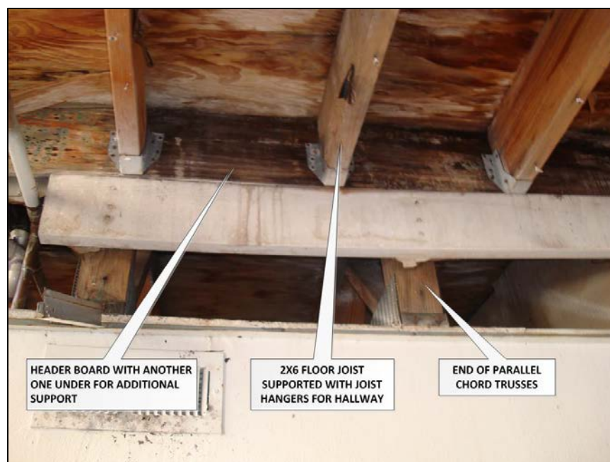
Photo 2. Close-up detail of hallway support construction. (NIOSH Photo)
