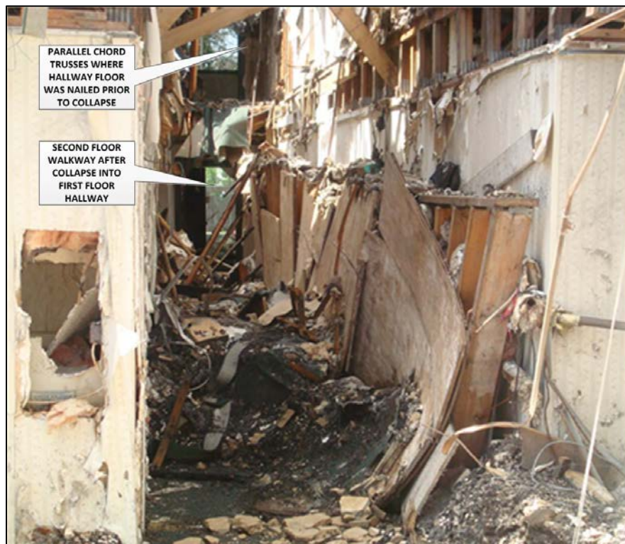
Photo 1. Hallway support construction in collapse area. (NIOSH Photo)
