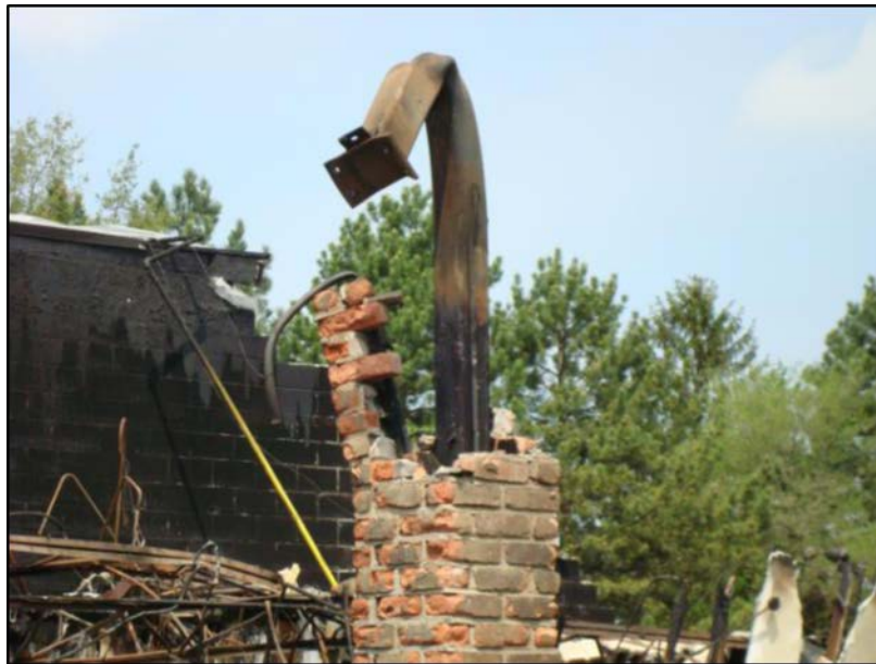
Photo 18. Tube Steel Column Failure- Roof Collapse. (Photo: NIOSH/ Analysis Diagram Courtesy of Buildingsonfire.com.)
