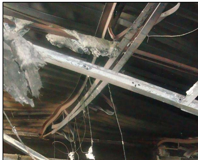
Photo 21. Detail of Truss Compromise and Roof Collapse.
