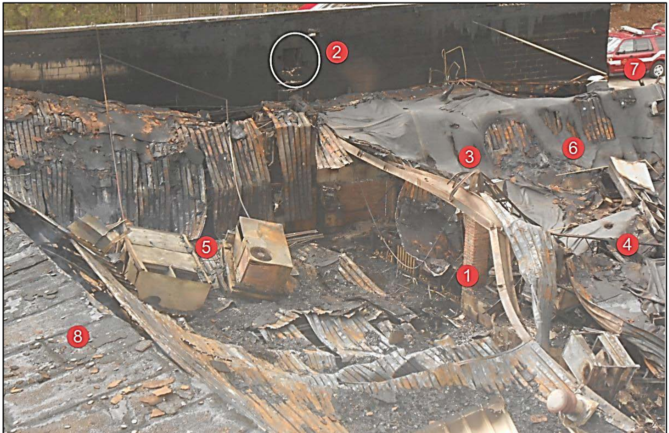
Photo 15. Pool Hall Roof Diaphragm Collapse –Charlie Wall and Delta Corner.
