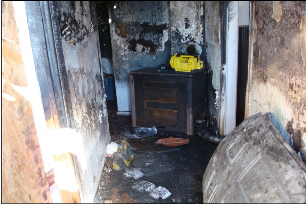
Photo 3. Hallway in which victim was operating prior to incident. Note the space heater that the victim was near when he yelled for help and the metal door that had been attached to the doorway in Photo 4 to the covered porch and was warped by the heat. (NIOSH Photo)
