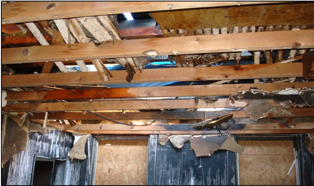
Photo 1. Second floor ceiling has multiple layers – drywall, 2 x 4 joists, lathe (subflooring), and 2 x 6 joists covered by OSB. (NIOSH Photo)
