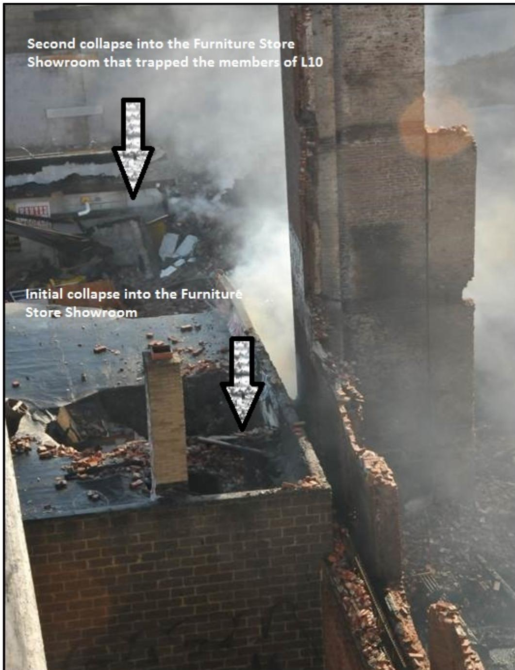
**Photo 13. Post collapse photo of furniture showroom roof showing the two holes made by the two different wall collapses.**
