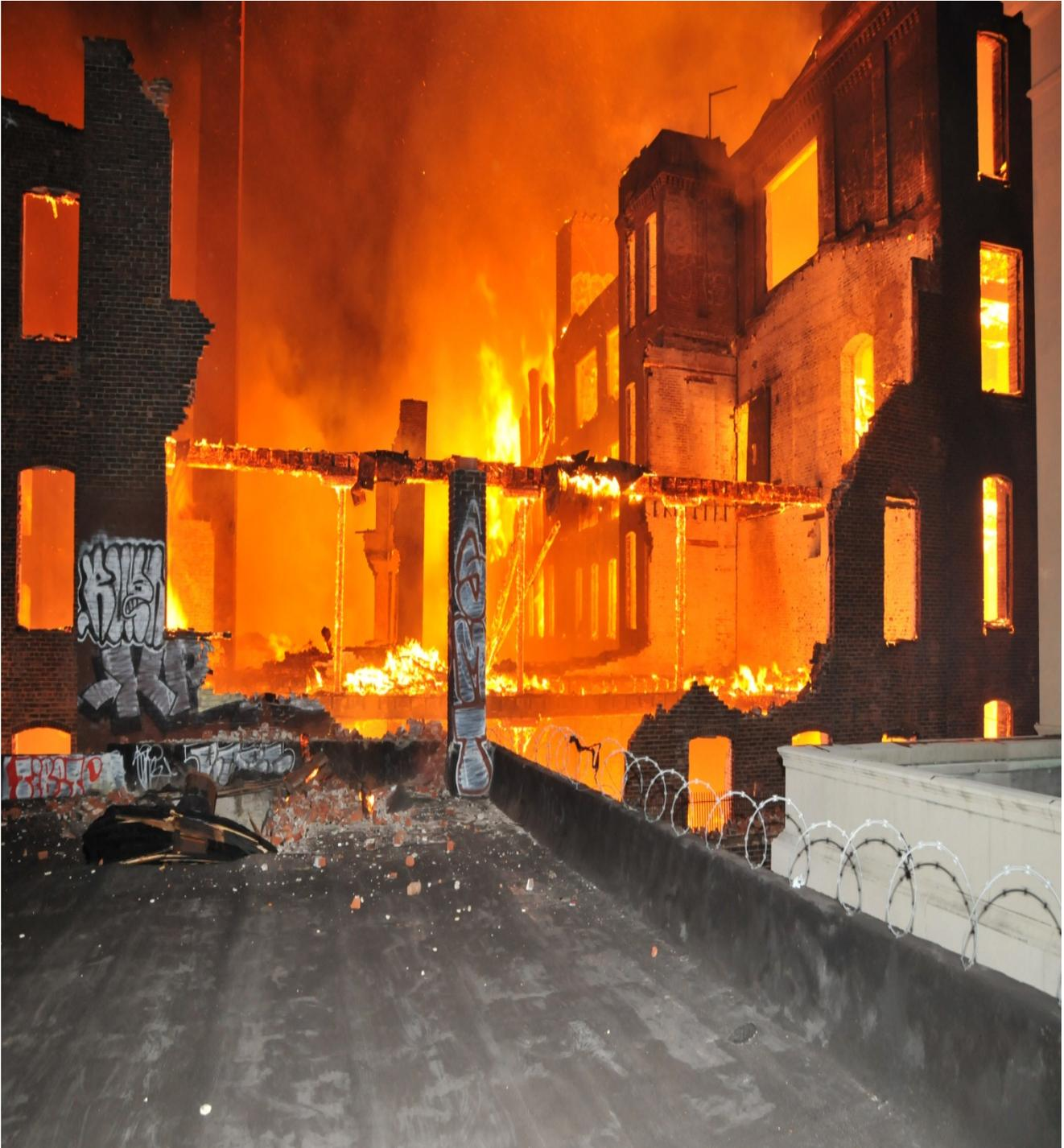
**Photo 12. Roof of the furniture showroom showing damage from a partial wall collapse that started the original fire inside the furniture showroom. (Photo courtesy of fire department.)**
