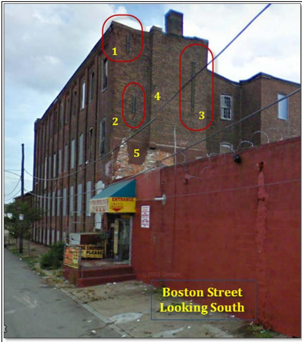
**Photo 4. Wall collapse indicators of north perimeter of Building #2, Side A exposure.**
