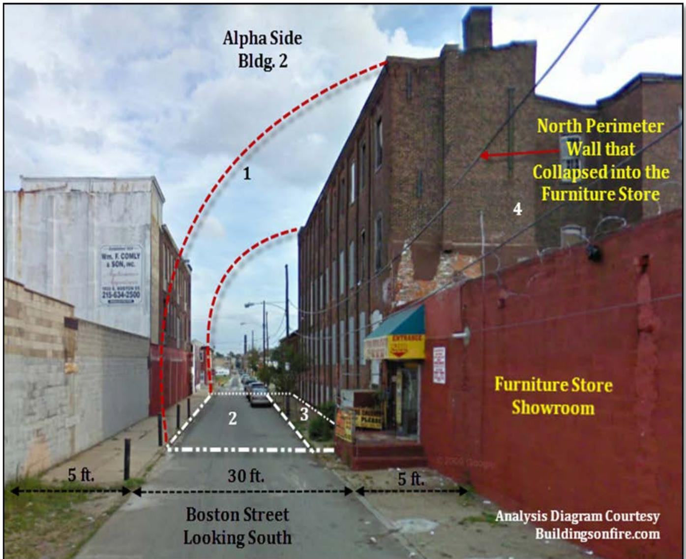
**Photo 7. Alpha Side –Wall Collapse Zones**
