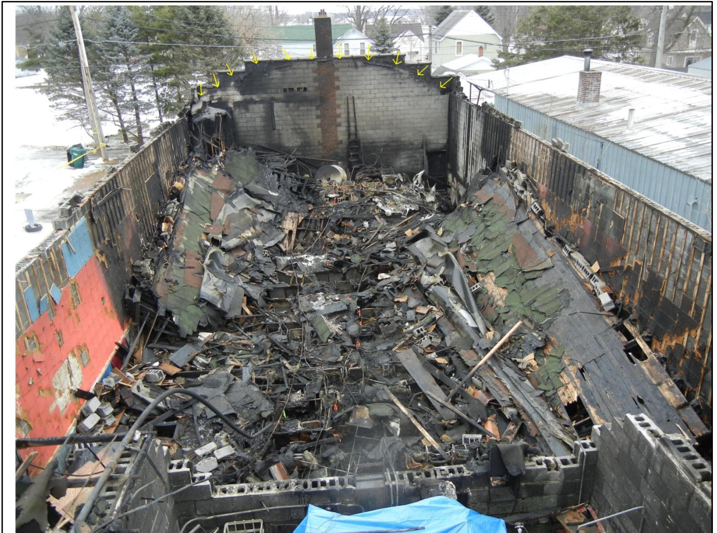
Photo 3. Photo taken from an aerial lift on the A-side of the structure showing the expansive area that the bowstring roof covered. Note the smoked dome outline, indicated by yellow arrows, on the far wall (C-side), indicating the location and span of the bowstring roof. (Photo courtesy of state of WI.)
