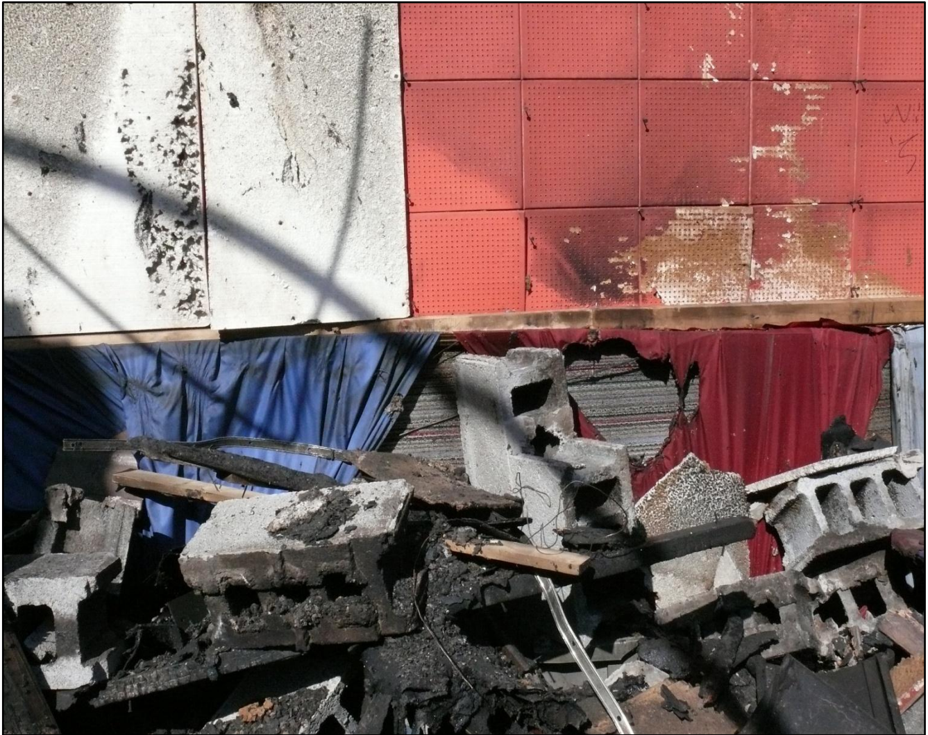
Photo 4. Interior auditorium walls, showing peg board, sound insulation, and wall curtains within the auditorium.
