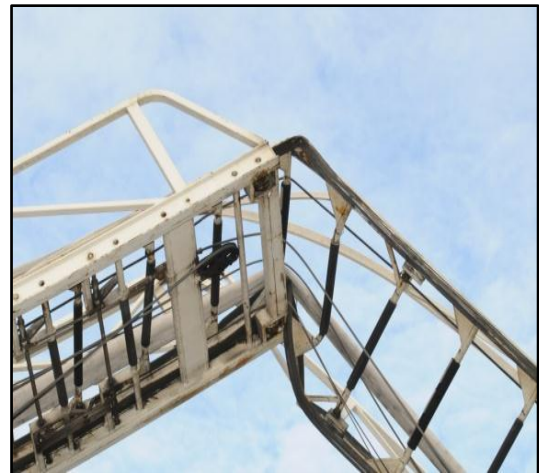
Photo 6. Structural failure occurred at end of the ladder bed section. (Courtesy of the Fire Department)
