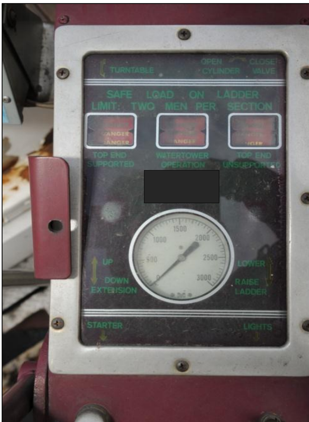
Photo 4. Three message windows displaying “Danger” (Photo taken after collapse, courtesy of the Fire Department)
