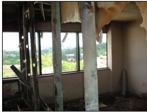
Photo 3. Interior studs of east wall of the fire room that the E1 fire fighter went through to get to the T1 platform at the window. (NIOSH photo)
