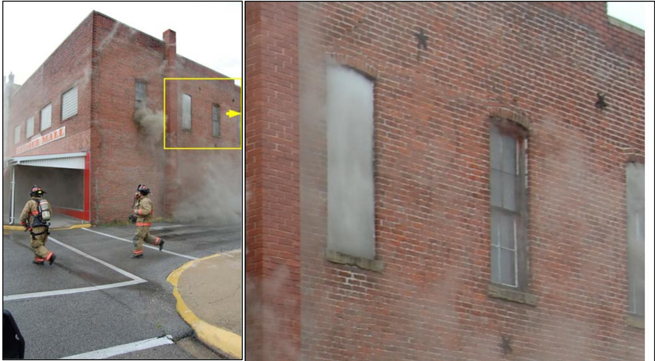
Photo 2 (left) and Photo 3 (enlarged – on right). Photos show star-shaped anchor plates located on the D-side wall in the area that collapsed, injuring the Victim. (Photo 2 courtesy of the local newspaper. Photo 3 edited by NIOSH)
