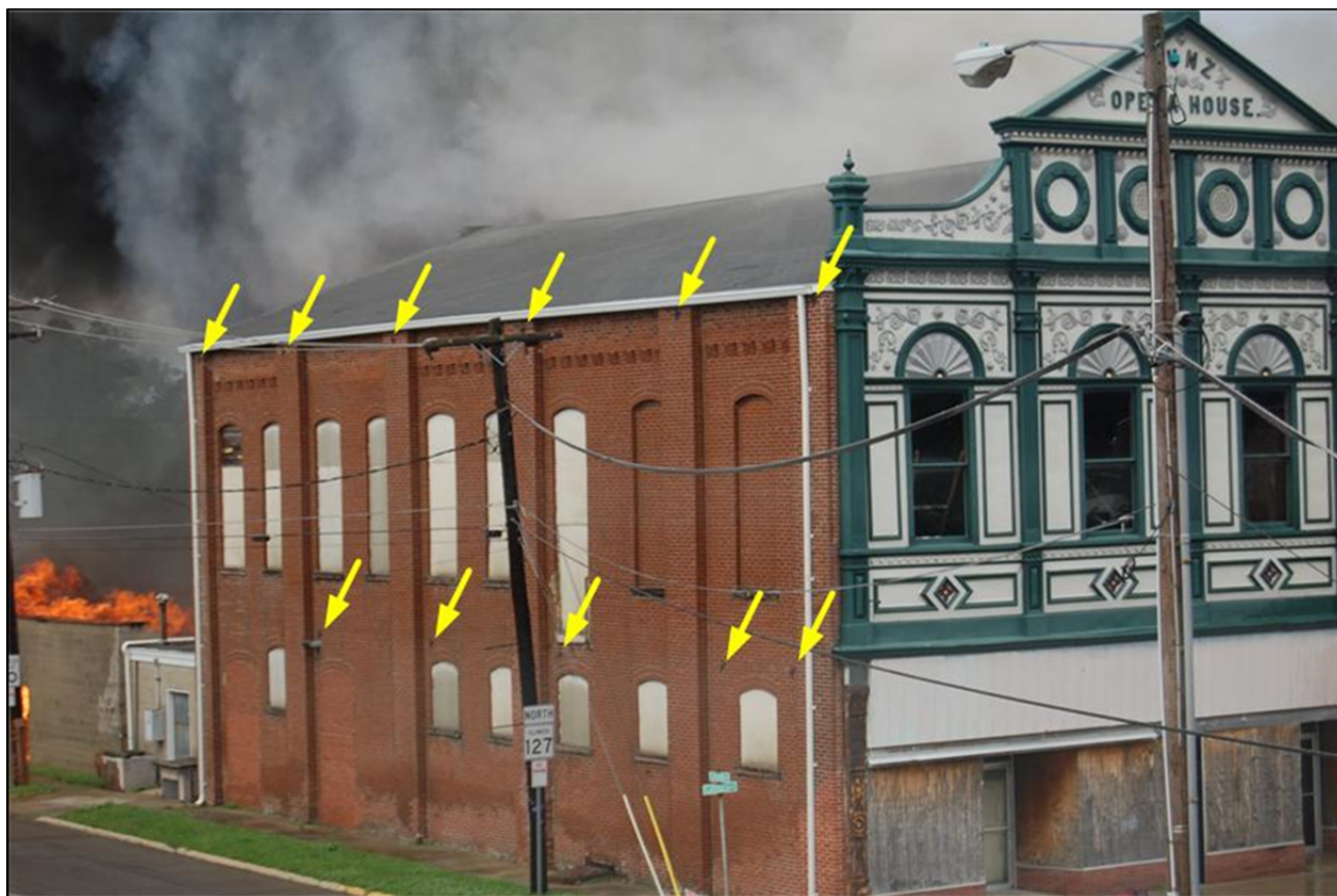
Photo 1. Arrows mark locations where star-shaped anchor plates were located on the west-side of the theater building that was adjacent to the fire building. The anchor plates appear to have been attached to the ends of the heavy timber roof trusses supporting the roof and also to some of the second-floor joists. See Photo 4 and Photo 5 for more details.
