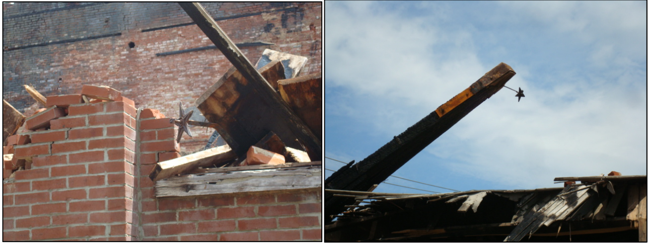
Photo 4 (left) and Photo 5 (right). Photo 4 shows star-shaped anchor plate attached to end of floor joist. Photo 5 shows star-shaped anchor plate attached to end of heavy timber roof truss. Both photos are of the theater adjacent to the fire structure. (Photos courtesy of the local newspaper)
