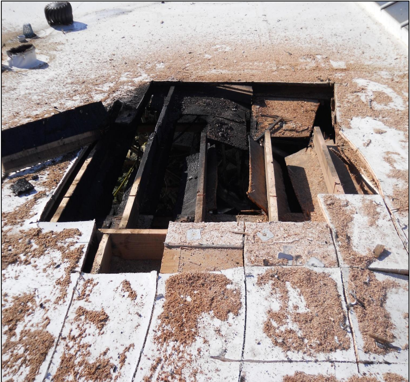
Photo 2. Photo shows roof construction and materials. Photo shows ventilation hole cut above the collapse area by the fire department the night of the incident.
