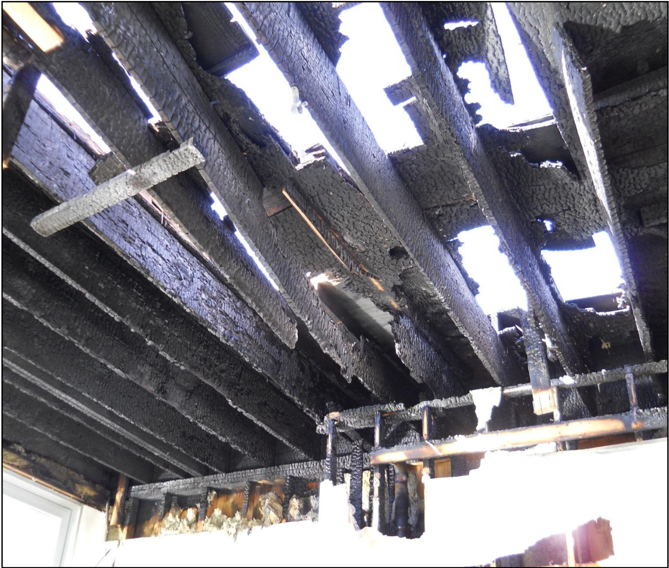
Photo 6. Photo shows void spaces between rafters. (Photo courtesy of mutual aid fire department.)
