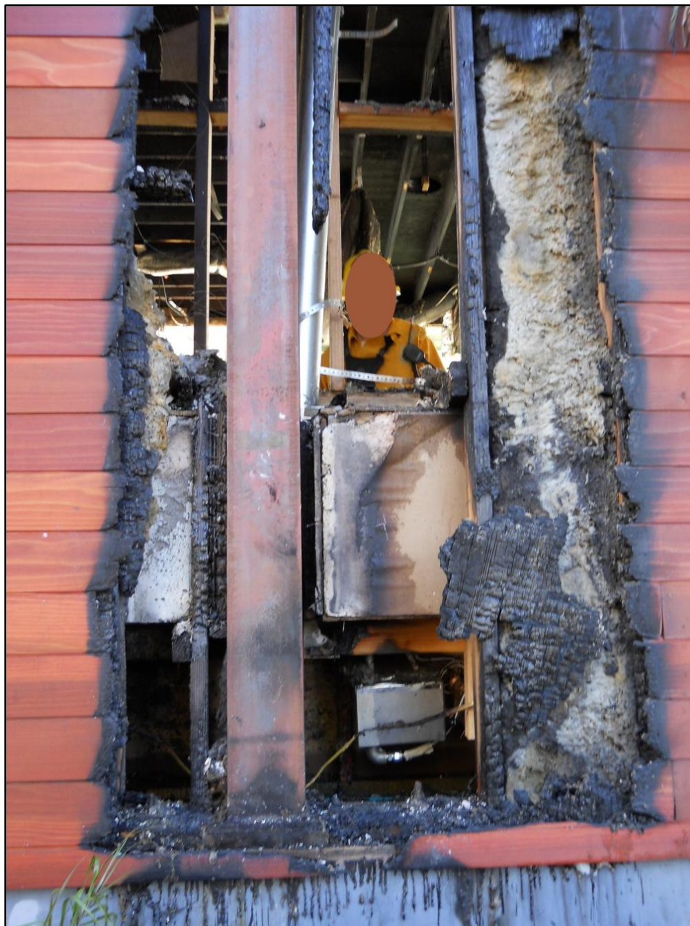
Photo 11. D-side exposure wall that was first observed showing fire by arriving units. Void space directly below fire place shows control box and charring to the combustible wood members. (Photo courtesy of mutual aid fire department.)
