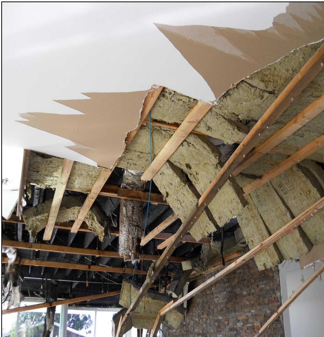
Photo 5. Photo shows ceiling construction of the drop ceiling where the collapsed occurred. (Photo courtesy of mutual aid fire department.)
