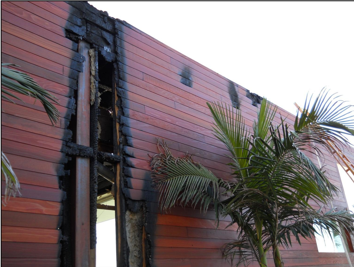
Photo 9. Photo shows burn pattern where fire was first observed by first arriving units. Photo taken after the incident was under control. (Photo courtesy of mutual aid fire department.)
