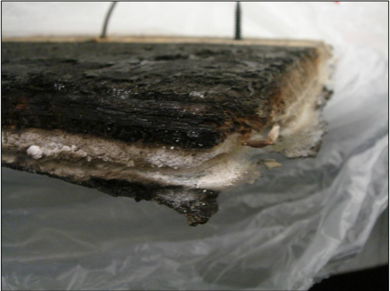
Photo 3. Photo shows the layers associated with constructing the home's roof membrane. (NIOSH photo.)
