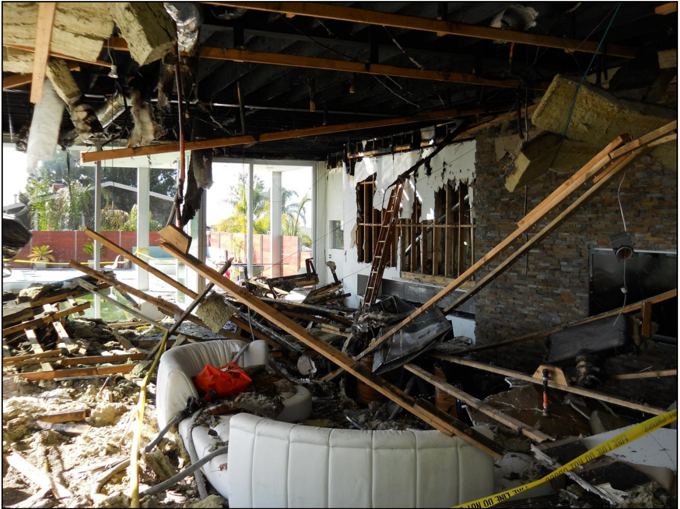
Photo 10. Photo shows the span of ceiling and debris that collapsed onto the interior fire fighters. (Photo courtesy of mutual aid fire department.)
