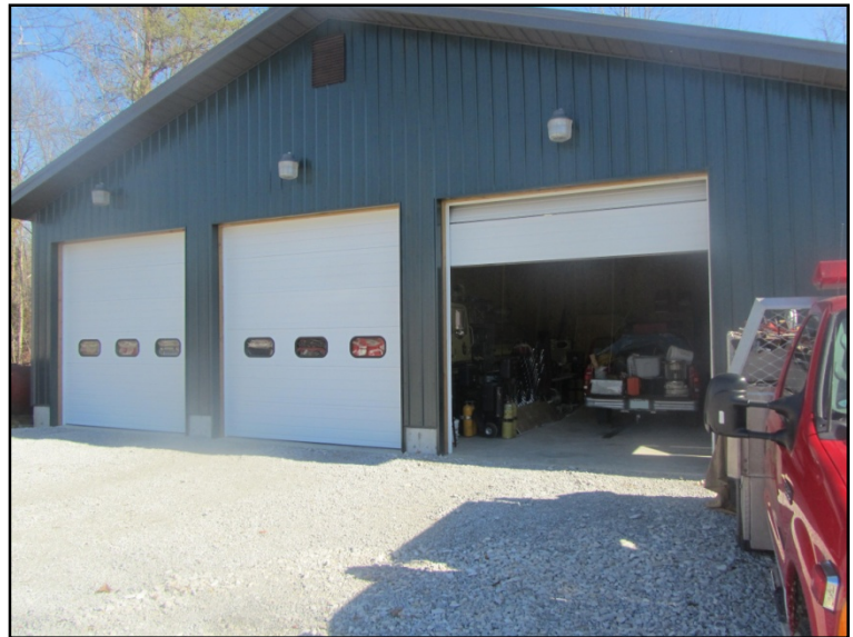
Open overhead door showing the vehicle and bay where the incident occurred four days prior.
