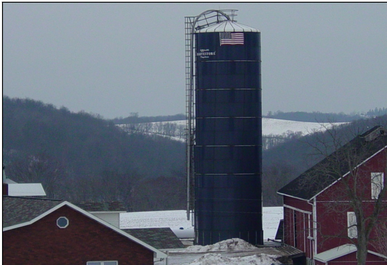
Photo 2. Oxygen limiting silo. This type of silo is distinguished by the flat or the slight-pitch to the roof, the lack of unloading doors along the length of the silo and the lack of a chute. (NIOSH Photo)
