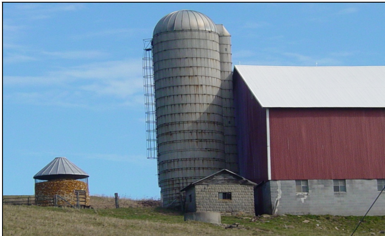
Photo 1. Conventional silo. This type of silo is distinguished by the round-domed top and the enclosed unloading chute seen on the right side of the silo, adjacent to the barn. (NIOSH Photo)
