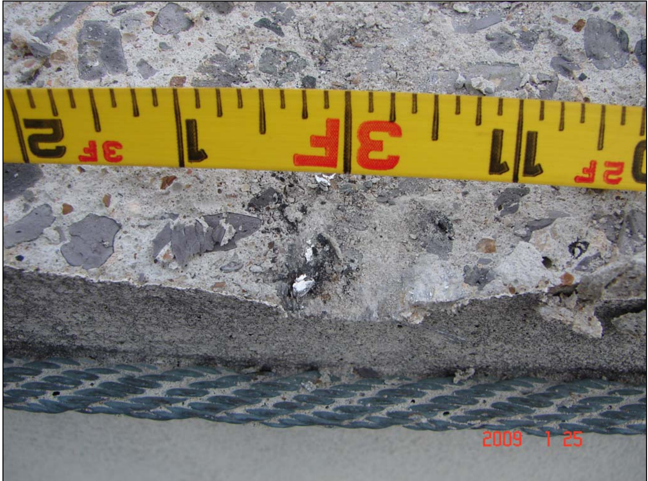
Photo 8. Slivers of metal visible in the gouge on parapet wall. Photo taken immediately after the incident by police detectives. Photo courtesy of police department
