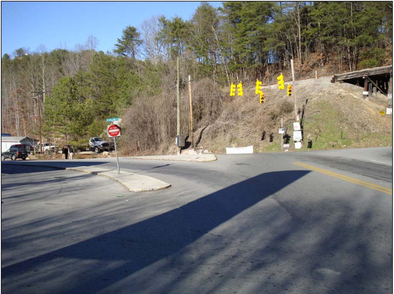
Photo 3. Intersection grade. Note the grade change of the intersecting roadway which would cause a vehicle to lean significantly to the right while making a left turn.
