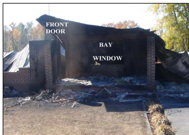
Photo 4. Incident scene after rekindle and collapse showing the front door and bay window. (NIOSH photo)
