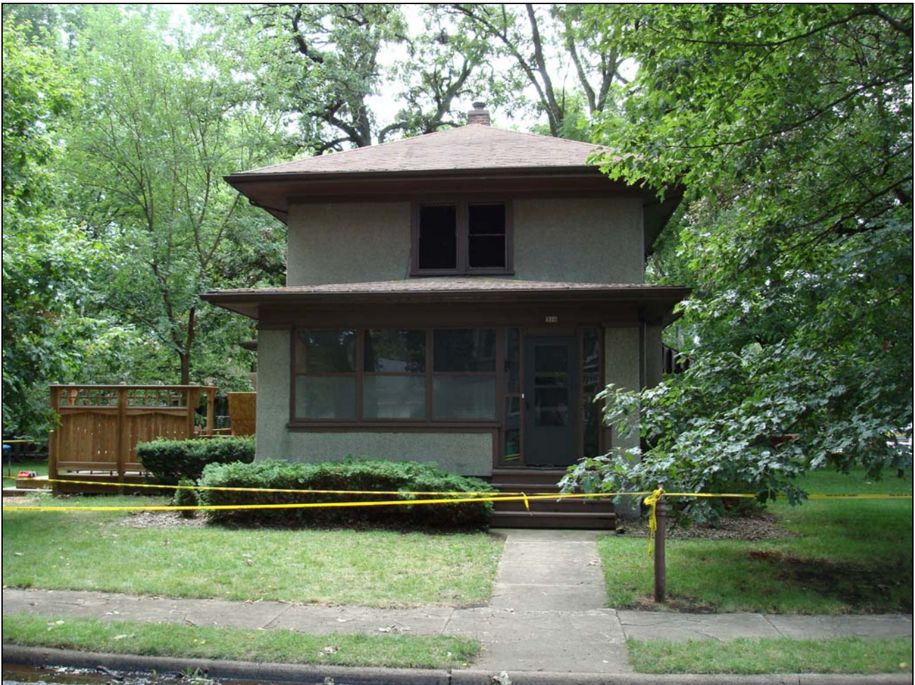
Photo 1. View of fire structure A-side and B-side deck. (NIOSH Photo)
