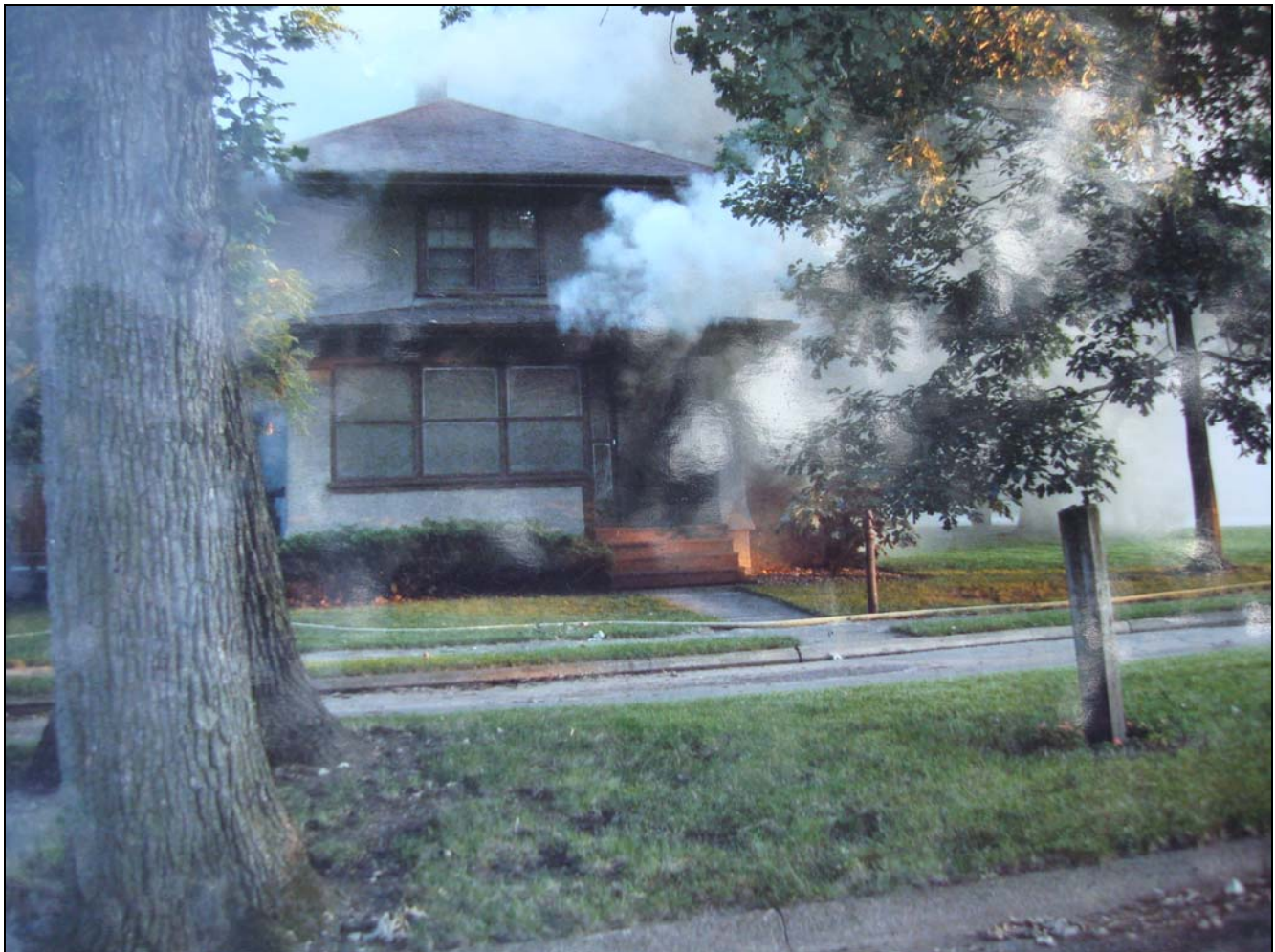
Photo 2. View of fire structure upon fire department's arrival. (Courtesy of fire department)
