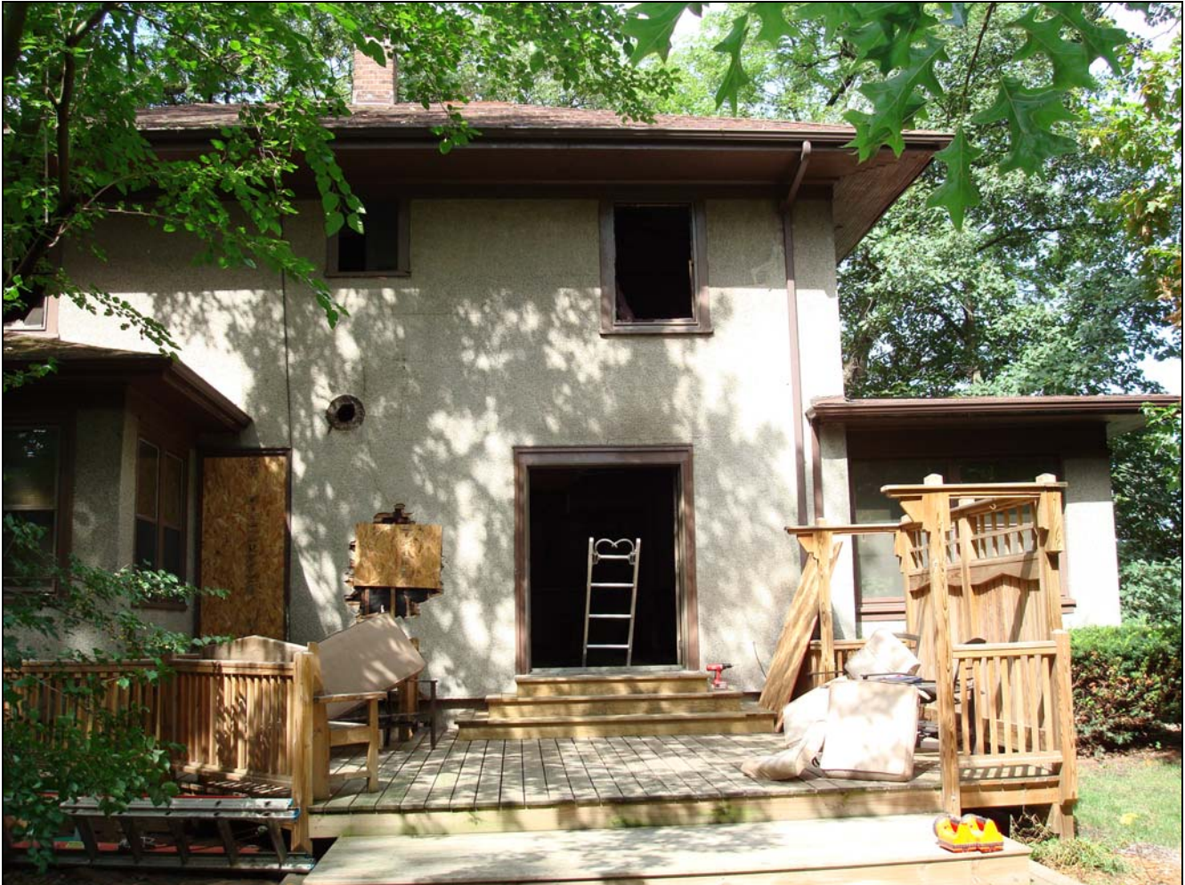
Photo 3. View of fire structure from the B-side deck and approximate placement of ladder when the victim was recovered. (NIOSH Photo)
