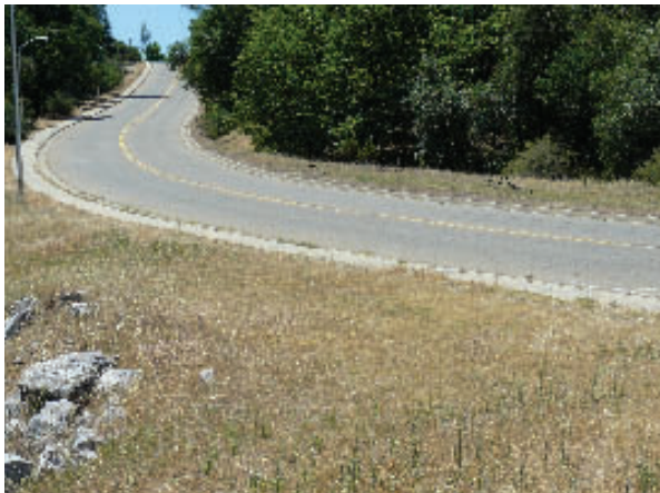
Photo 2. Steep section of the route
