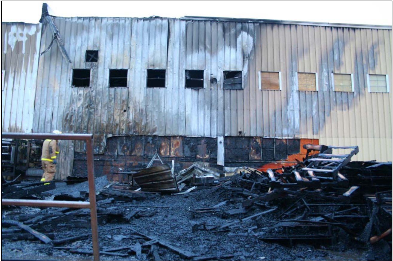
Photo 9. Photo shows the remains of the fuel load on the loading dock following the fire. (Photo courtesy of Matt Skrekla.)
