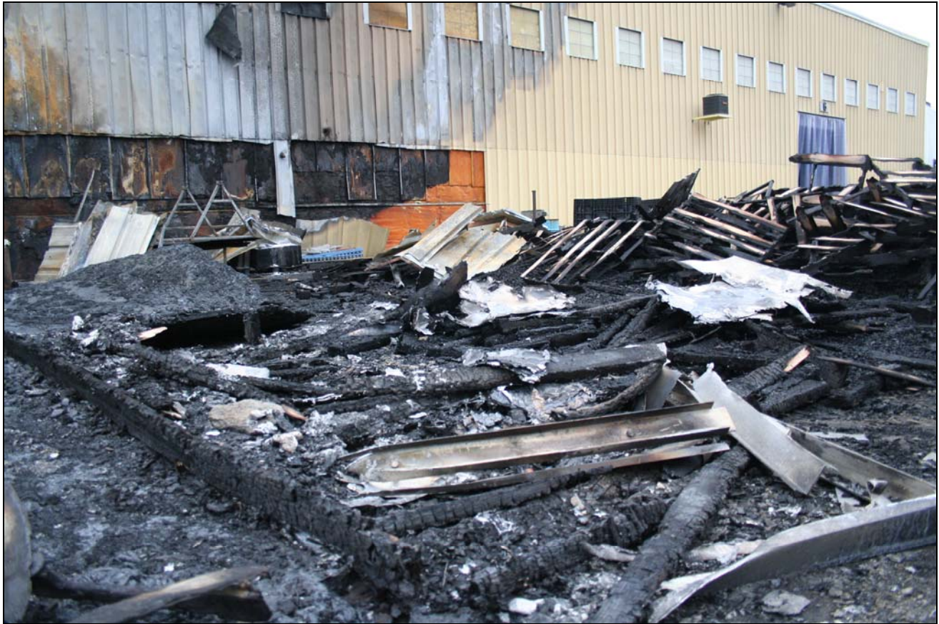
Photo 7. Loading dock area immediately after fire. Note the fuel load present on the loading dock consisting of wooden and molded-plastic pallets. (Photo courtesy of Matt Skrekla.)
