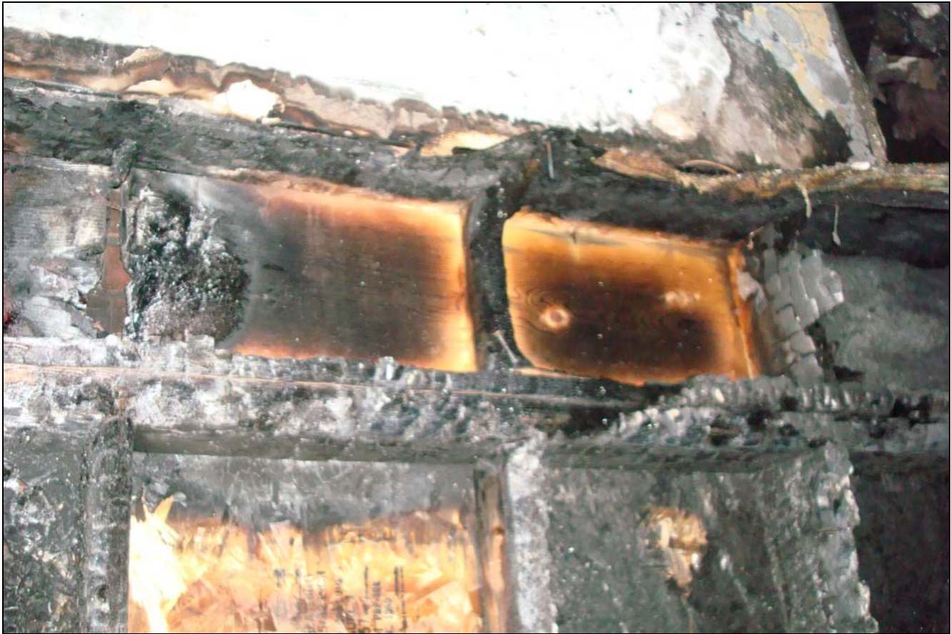
Photo 6. Burned away floor joists above the small cedar closet along the C-side wall. (NIOSH photo)
