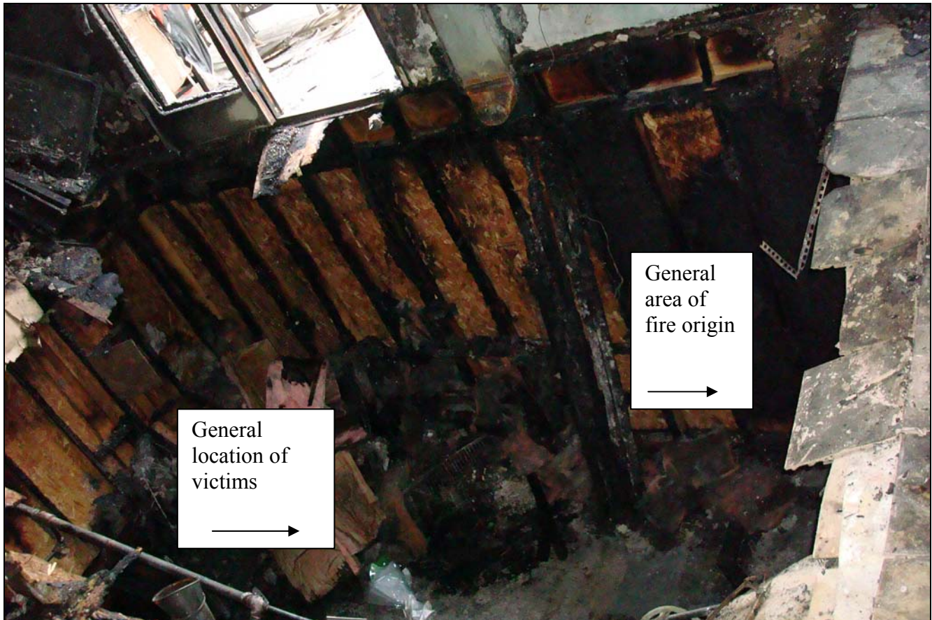
Photo 4. Collapsed section of floor the victims crawled across and the approximate location of their bodies in the basement. (NIOSH photo)
