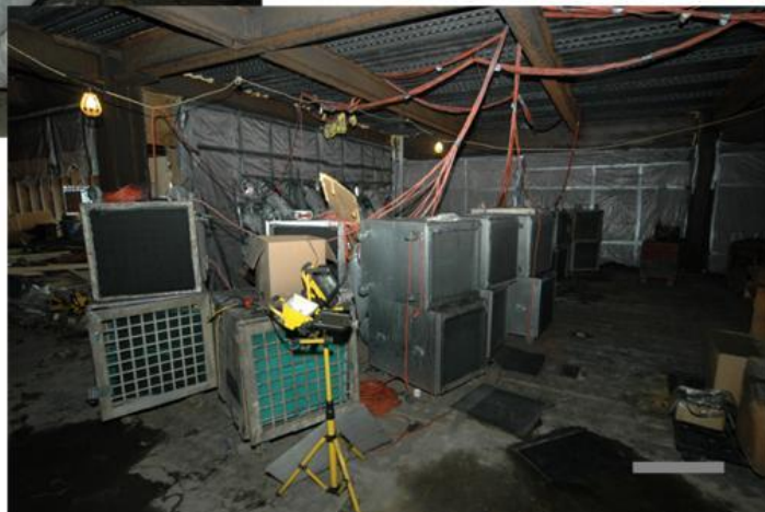
Photo 5. Plastic sheeting, ductwork and fans used for asbestos abatement. (Photos courtesy of fire department.)
