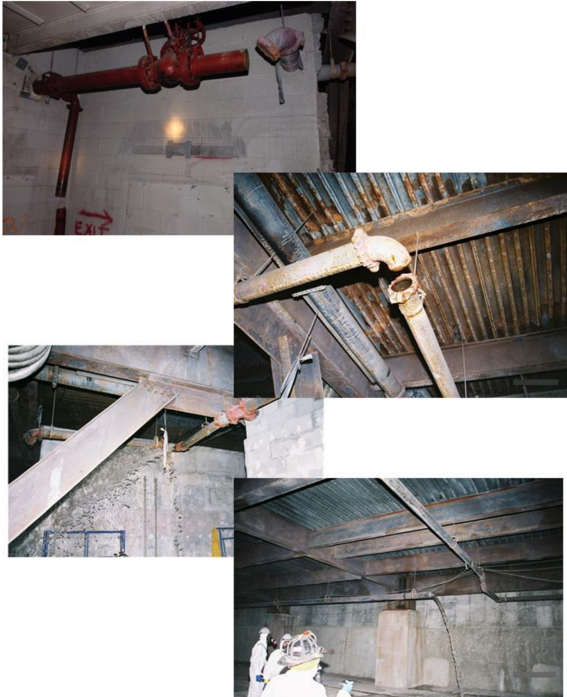
Photo 4. Standpipe system was inoperable due to missing sections of pipe. (Photos courtesy of fire department.)
